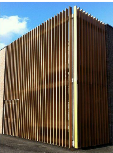
TIMBER BRISE SOLEIL
