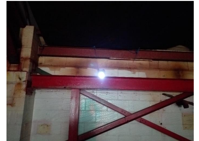
12 - Access point via wall pipe (Feature 7)
