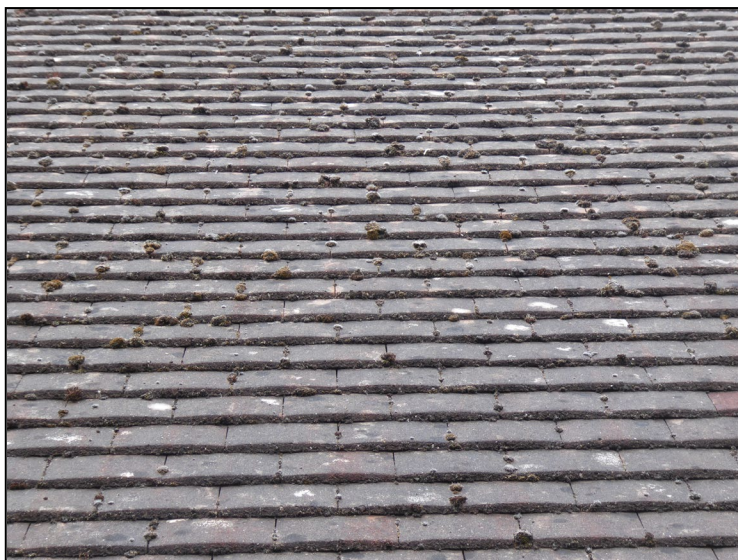
Figure 4. Well-fitting roof tiles. Garage at 6 Soane End, Emmer Green. 10.06.21
