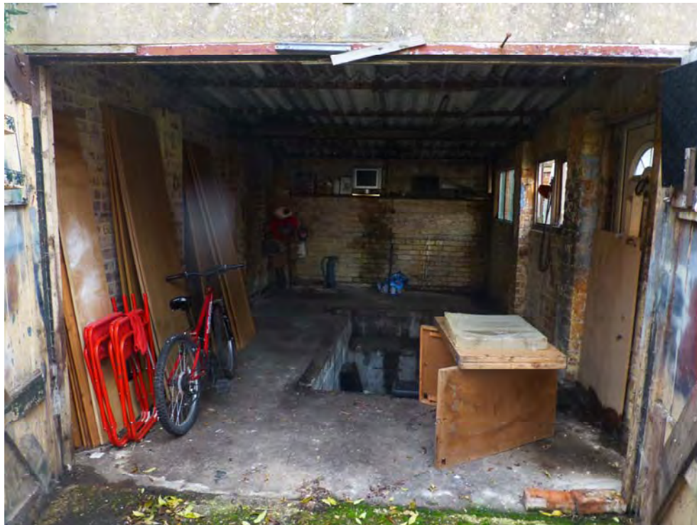
Photograph 7: An internal view of the garage unit.
