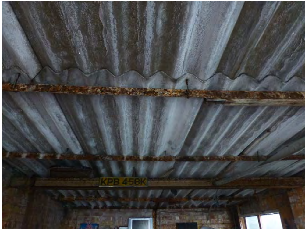
Photograph 11: A view of the roofing fabric showing corrugated cement bonded sheets – possibly containing asbestos fibre.
