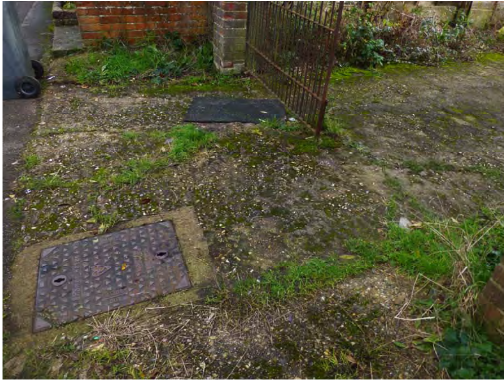
Photograph 3: A closer view of the concrete located at the front of the site. Note drainage covers indicating surface or foul water systems.
