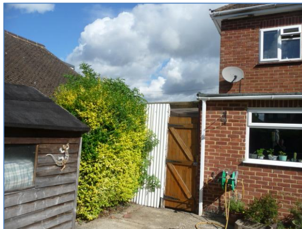
3. Side boundary to 45 Crescent Road taken from rear garden. Photo provided by the agent on 23/10/2020.
