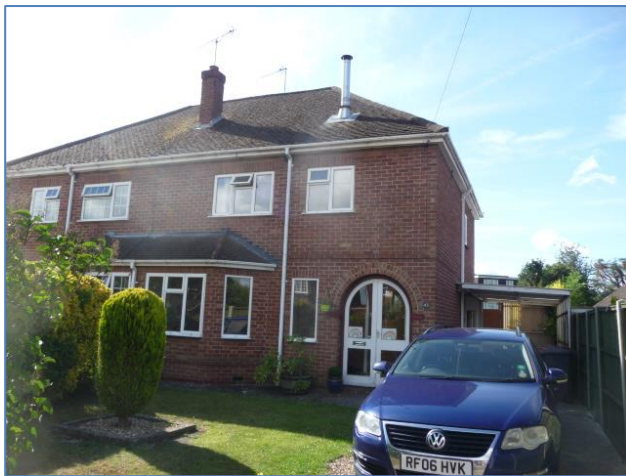
1. Rear of 43 Crescent Road. Photo provided by the agent on 23/10/2020.
