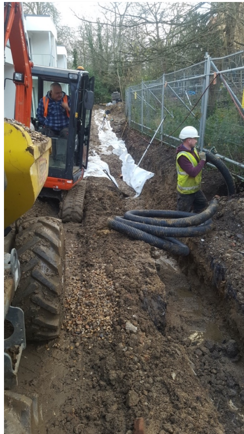
Figure 4. Common trench to north of tree protection fence within RPAs of 3029 and 3030, shows spur to lamp column opposite 3030 being installed
