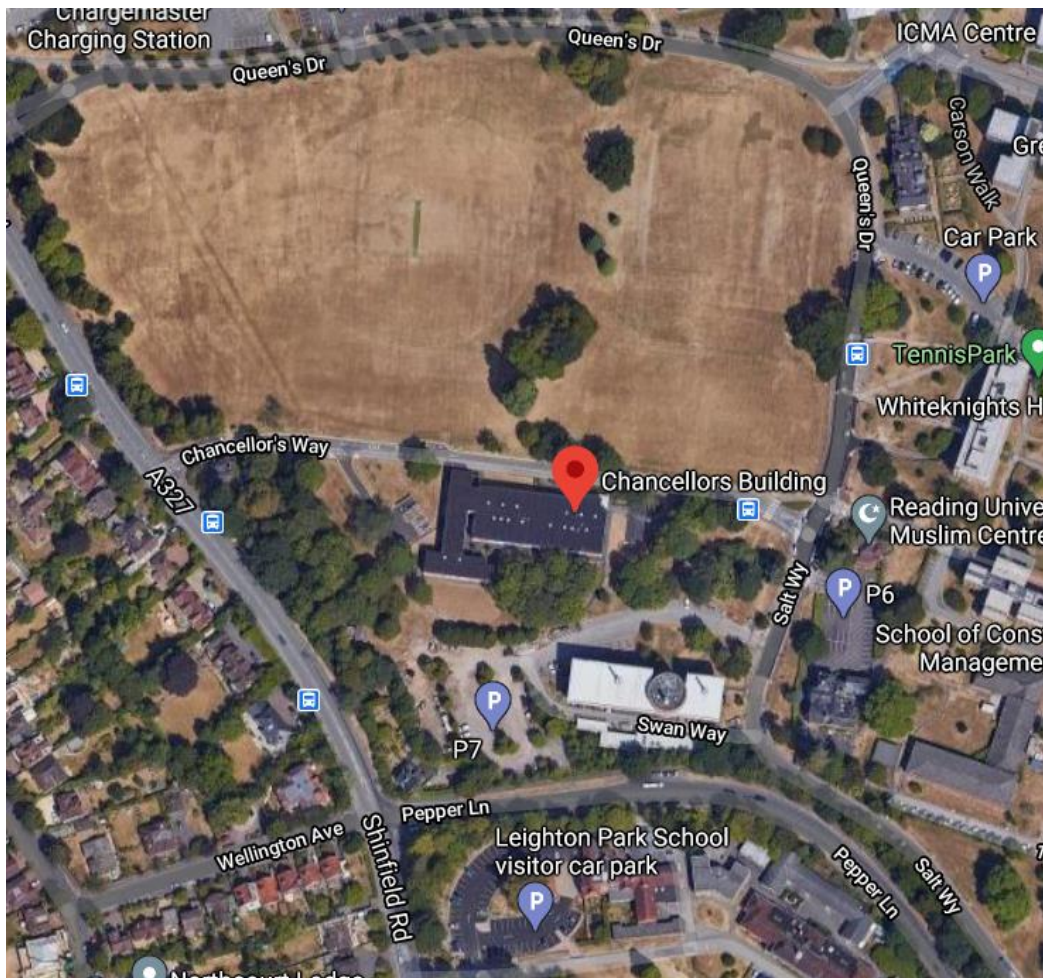
Image 1 – Aerial View of the Site
