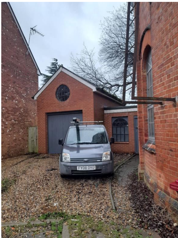
Photo 3 Looking towards the store.
