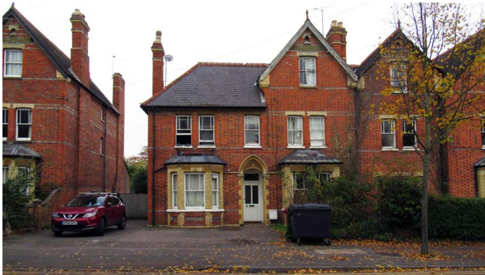
Fig.1: View of the front of 11 Addington Road
