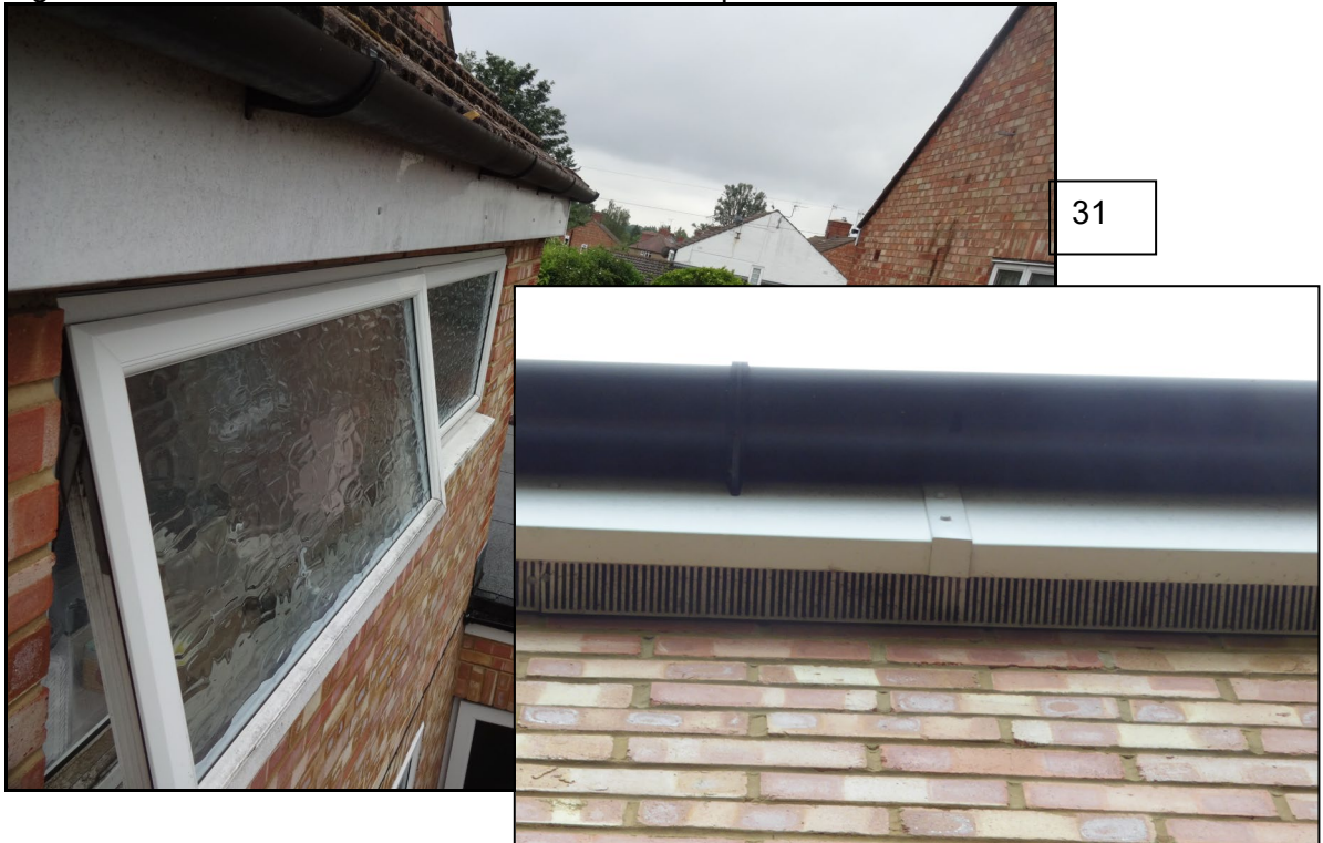
Figure 6. Sealed soffits and fascias. 31 & 33 Hilltop Road, Caversham. 28.06.21
