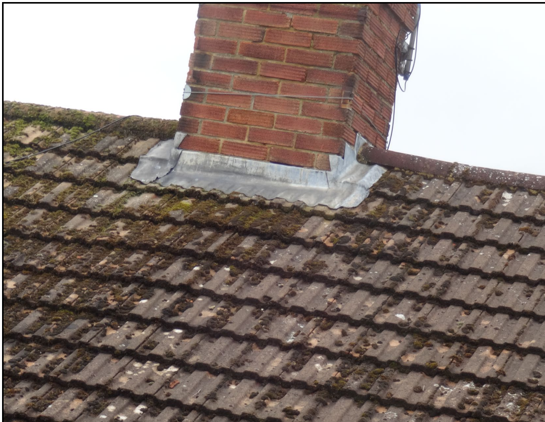
Figure 8. Flashing around shared chimney. 31 & 33 Hilltop Road, Caversham. 28.06.21
