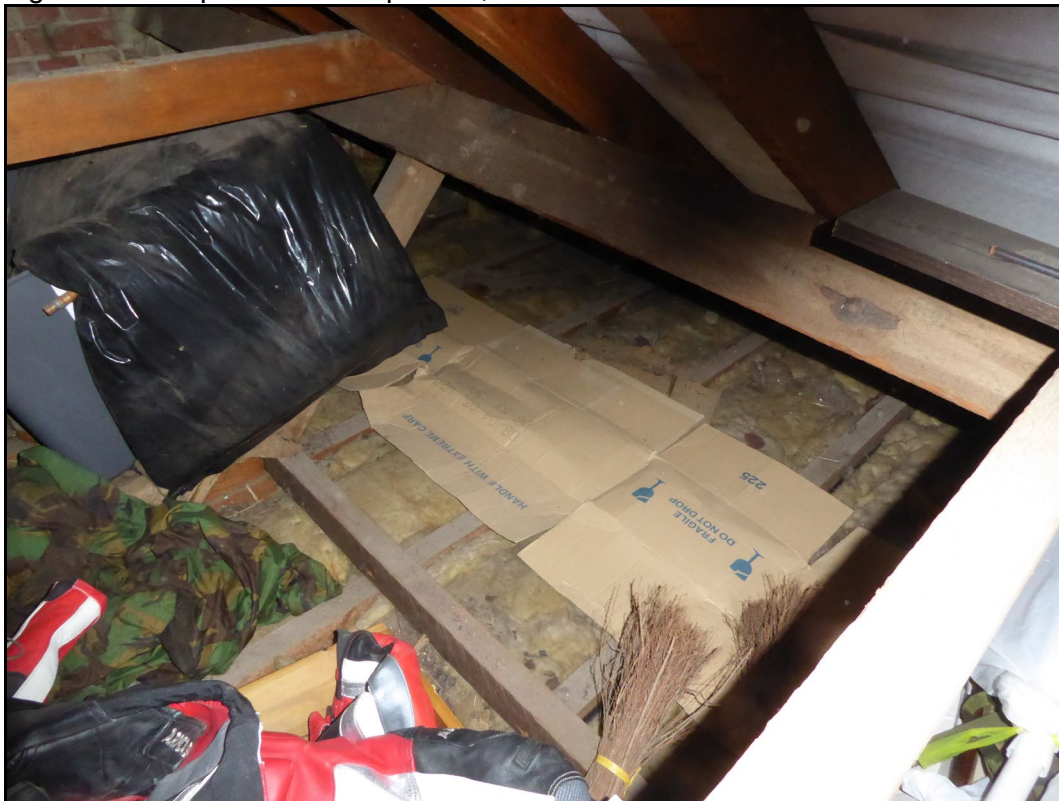
Figure 9. Loft space. 31 Hilltop Road, Caversham. 28.06.21
