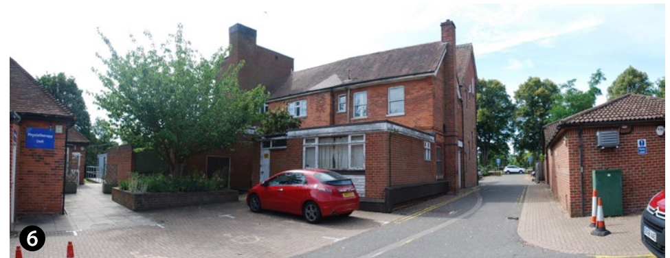
View west along the access road from the rear of Block One
