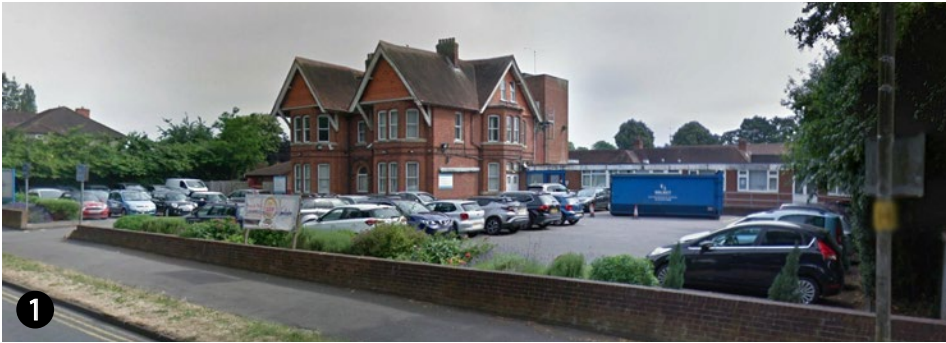
View north-east from Liebenrood Road, showing Block One and the car park
