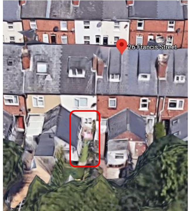
Fig 2. Existing rear elevation at 26 Francis Street (photograph provided by agent).
