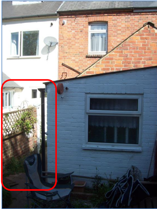
Fig 1. Existing rear elevation at 26 Francis Street (photograph provided by agent).
