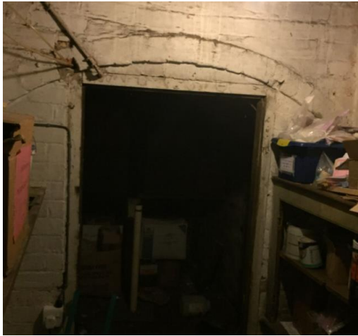
6. Original brick arch
