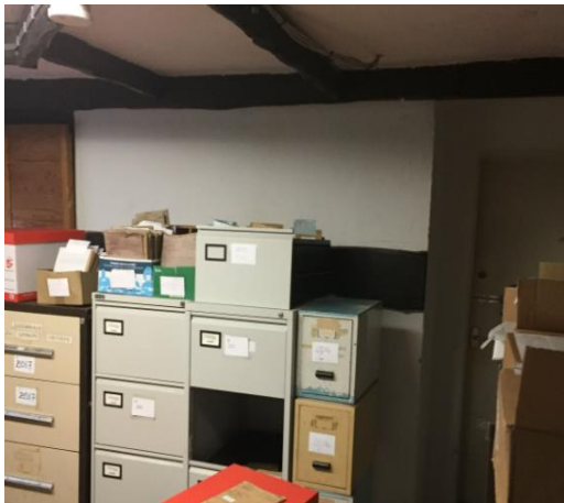
7. Timber beams in ceiling
