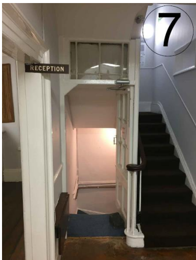
13. Ground to first floor stair to 165
