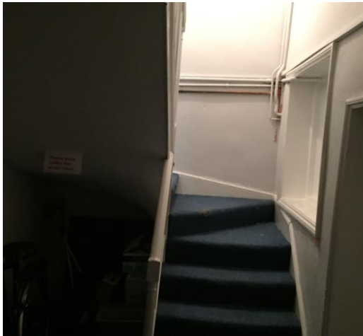
1. Stair with later treads and skirting
