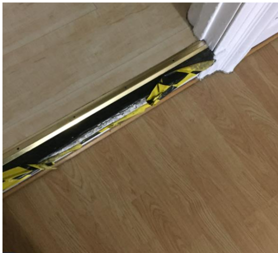
33 Change of floor surface
