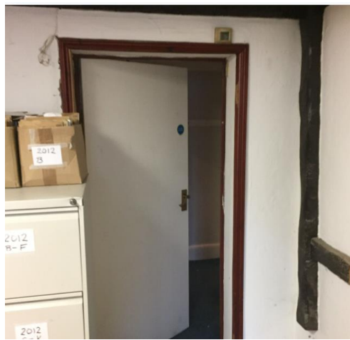
7. Imitation architrave and old/ new timber beams
