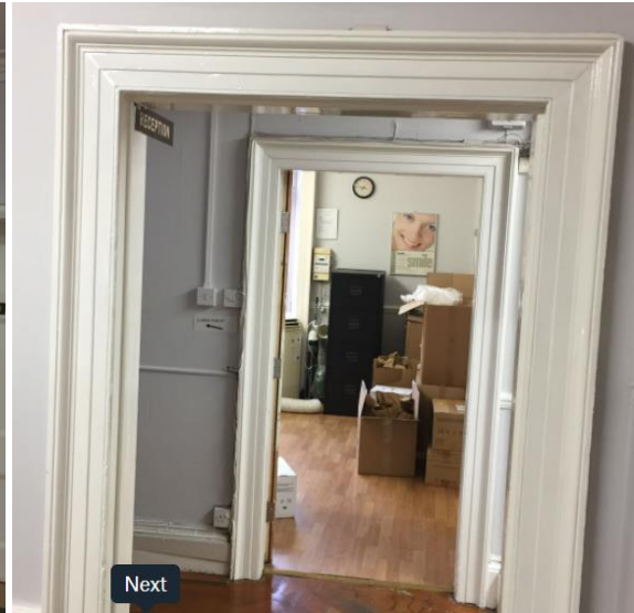
25 Matching architraves either side of landing
