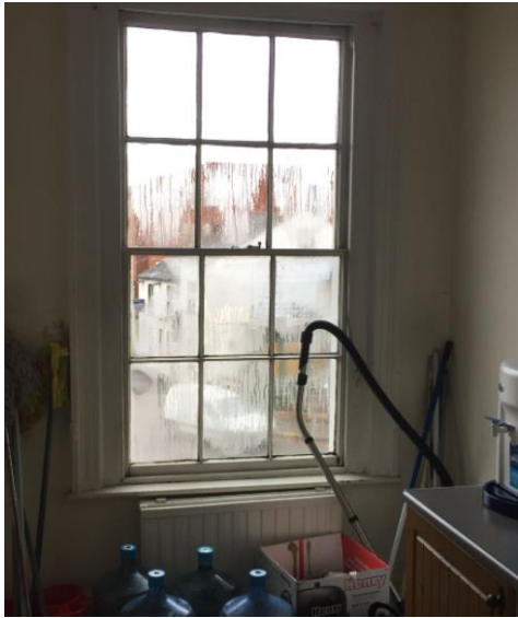
34 Sash window in kitchen
