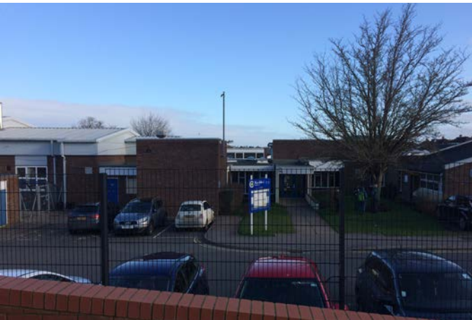
View of existing School entrance on site - western side
