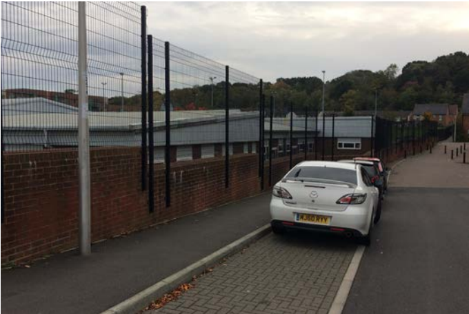
View of existing school from Deveron Drive to the north
