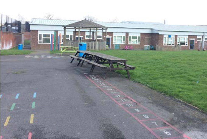
Views of existing western side of school and grounds from existing playground
