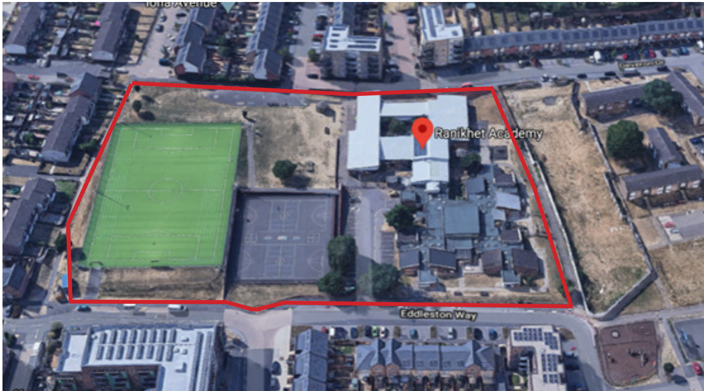
Aerial view of site from south
