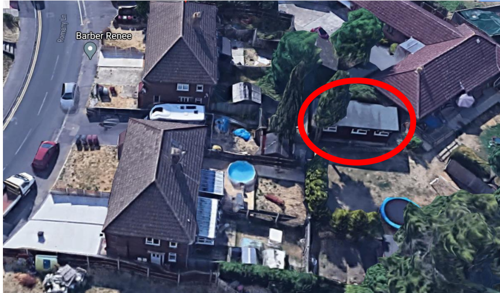
View of the studio/ annexe from above to give a greater perspective of the building in relation to surroundings. The building is highlighted with a red circle (Image: Google Maps)
