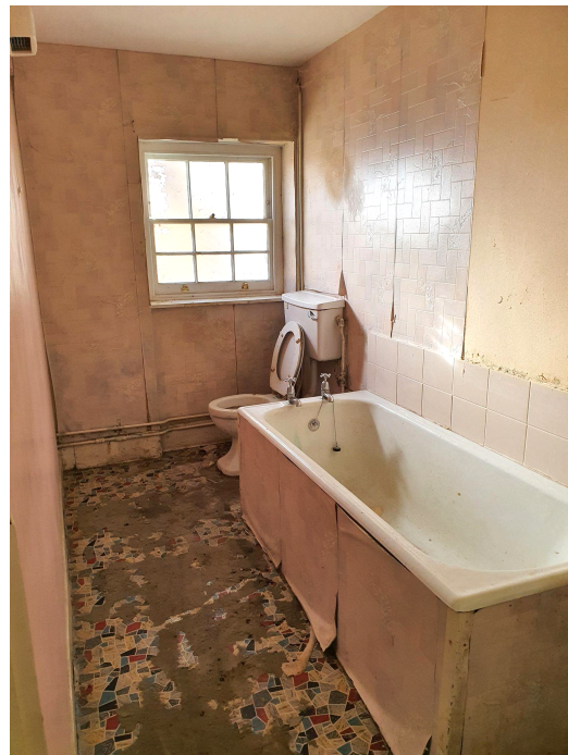
Figure 2: This photograph also shows the amount of natural light and the depth that it can reach in the lower ground floor room through the window. This photograph was also taken in July 2020 at 16:40.
