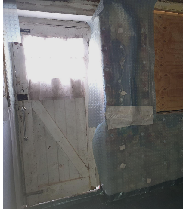
Figure 4: This photograph shows the front entrance door and how much daylight can reach in the lower ground floor room through the partially glazed door. This photograph was also taken in July 2020 at 16:40.
