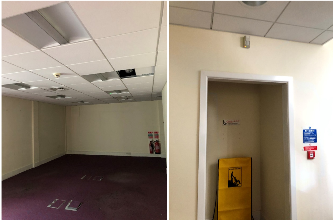
Stud walls, suspended ceilings, refuge and lift to be removed.
