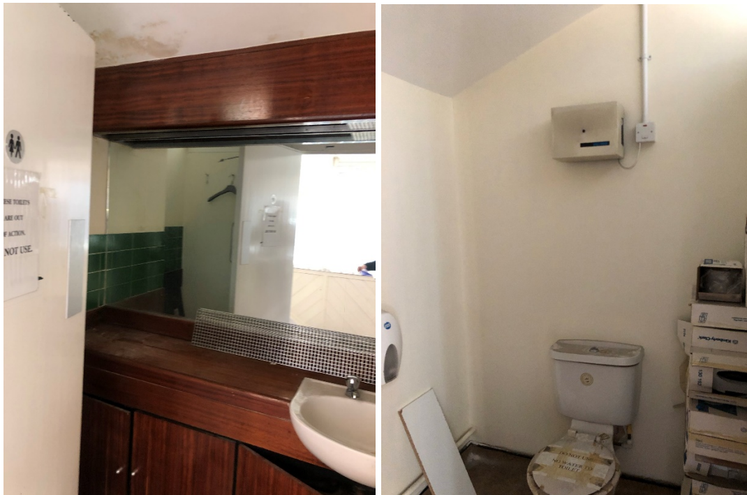
Existing toilets to be removed.
