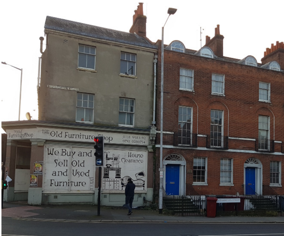
Front of No. 86 Southampton Street
