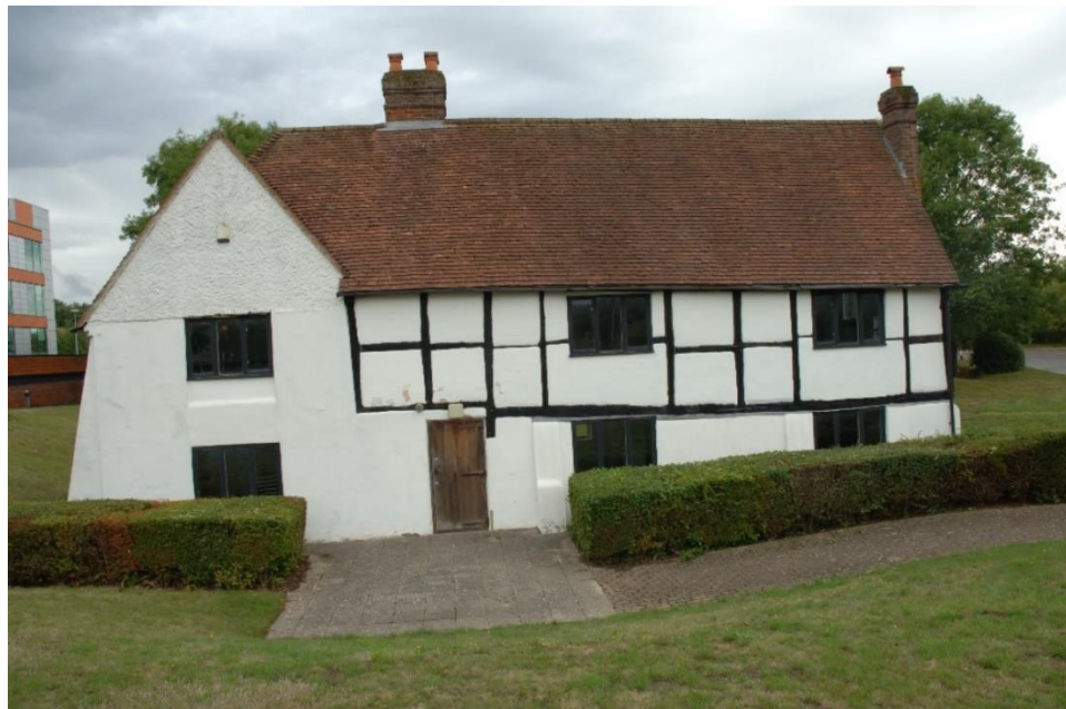
Figure 4.3 Old farmhouse building (building 3)
