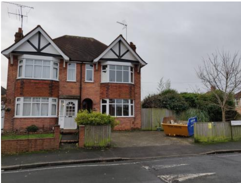
Photo 3. Taken from opposite number 41 Drayton Road. Due to the set back of the proposed two storey side extension being over 5m back from the front wall of the existing house, the extension would be barely visible from this position and would appear to be very subservient to the main dwelling.
