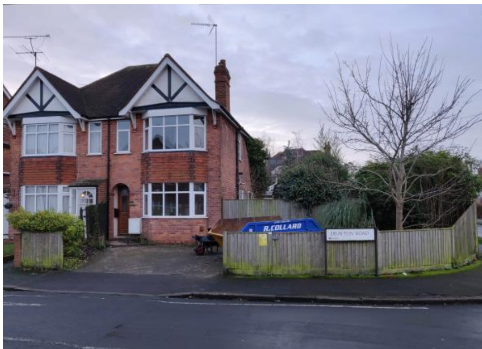
Photo 1. Taken from the opposite pavement, with the 1.9m high close boarded fence and hedging visible to the front.
