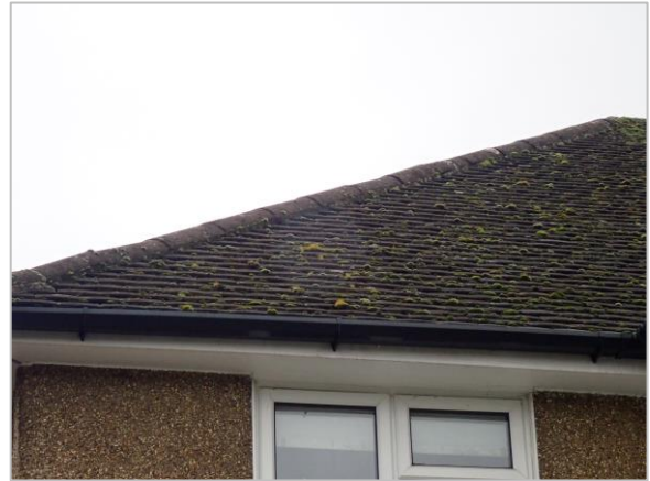
Photo 14 Roof tiles to front of house
