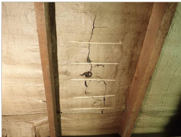
Photo 11 Repairs to underfelt
