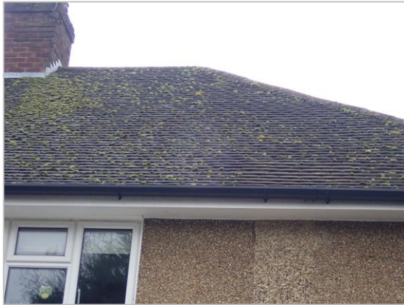
Photo 13 Roof tiles to rear of house
