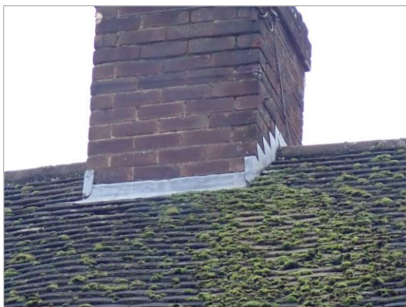
Photo 17 Chimney flashing
