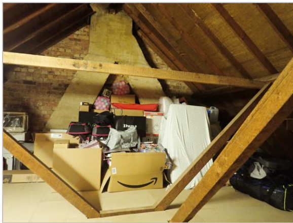
Photo 3 General conditions in main loft (northern partition wall)
