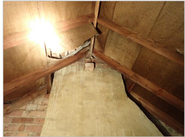
Photo 8 Top of chimney breast
