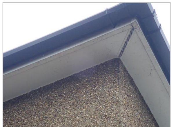
Photo 18 Soffit around south-west (rear) corner of house
