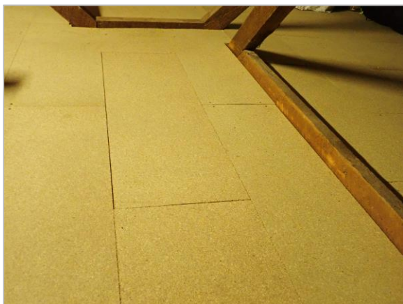
Photo 5 Main floor area of loft
