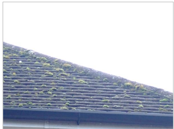
Photo 16 Hip ridge tiles in good condition
