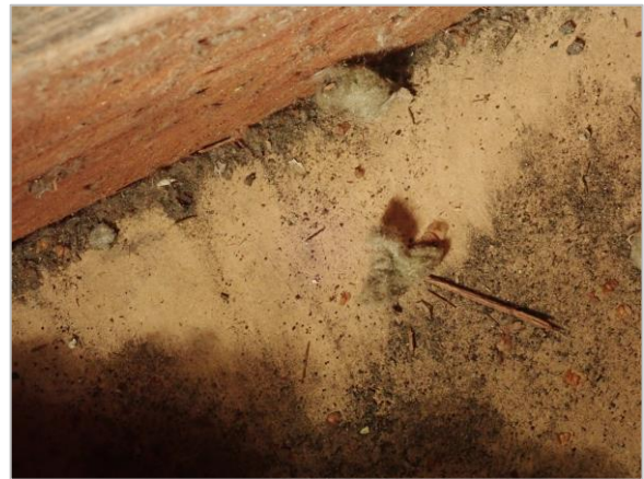
Photo 10 Spot check beneath insulation
