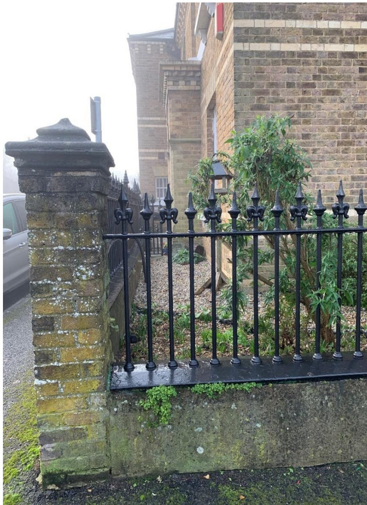
Close up of brick pier to be replicated
