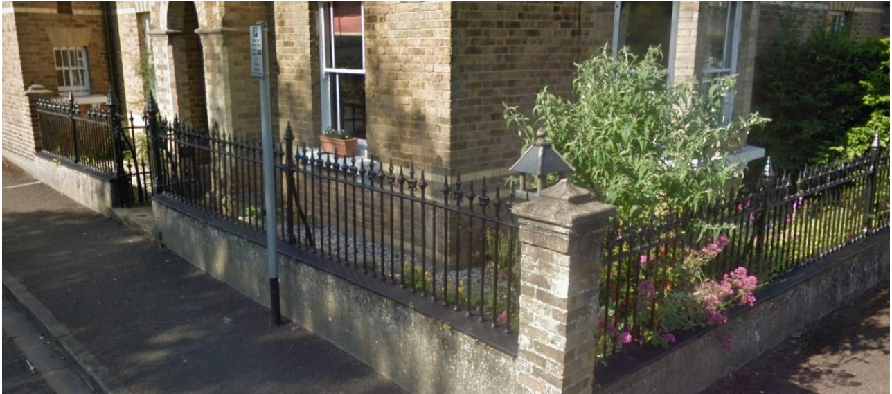
Existing railings of No.8 The Mount to be replicated
