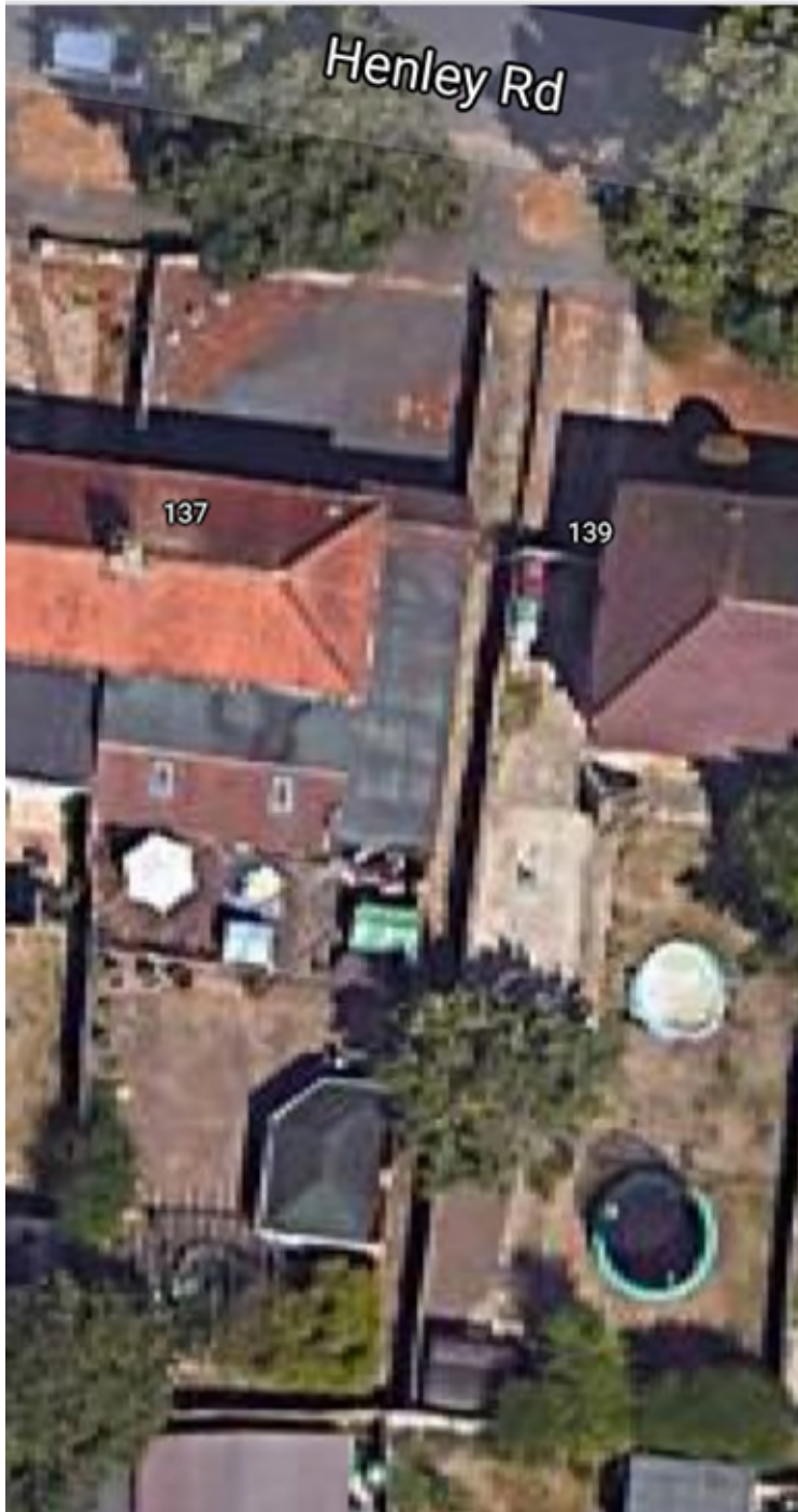
Picture 1 - No 137 of Henley Road is having a double storey side extension and rear extension with flat roof.
