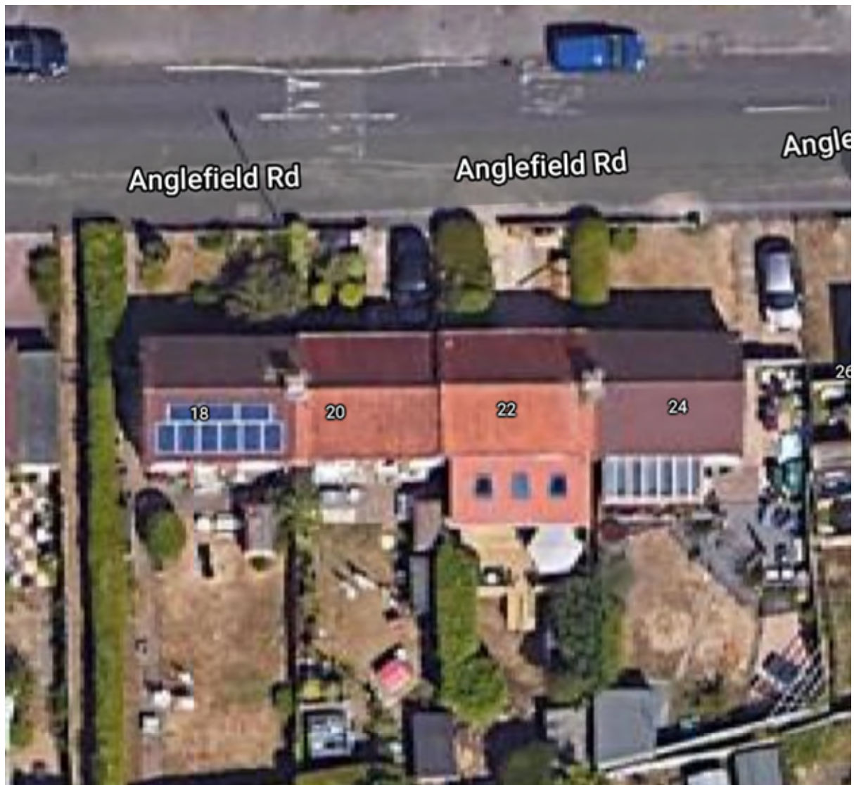
Picture 2- No 22, Angel field Road has a doble storey rear extension with flat roof
