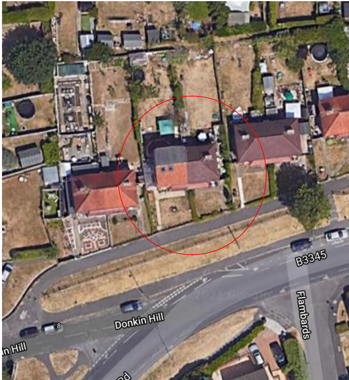
Picture 4 – House behind our house, loft converted with full dormer with flat roof
