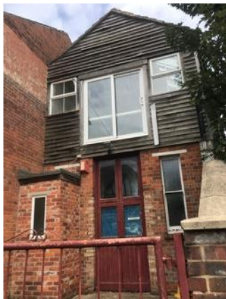
Photograph 1: West elevation of the building
