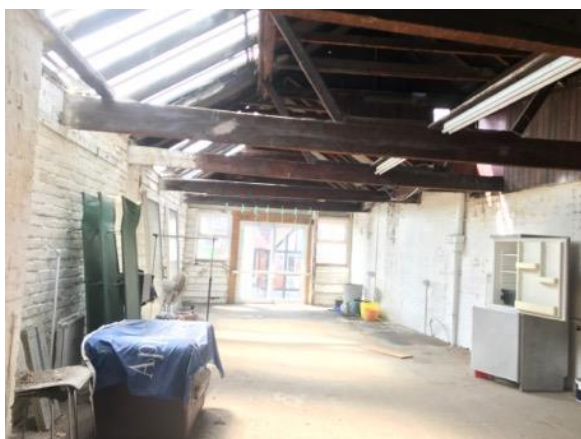
Photograph 9: Gap between interior brickwork and beams
