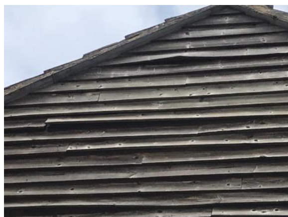
Photograph 4: Raised weatherboarding on the west elevation of the building
