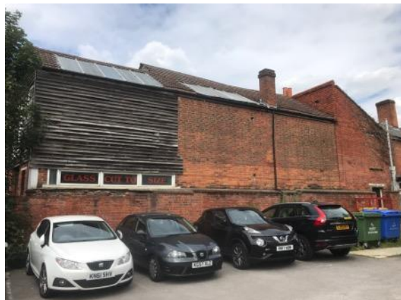
Photograph 2: South elevation of the building
