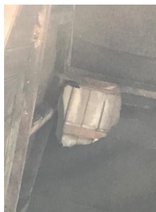
Photograph 10: Hole in roofing membrane
