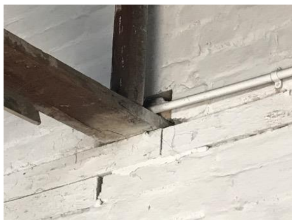
Photograph 9: Gap between interior brickwork and beams
