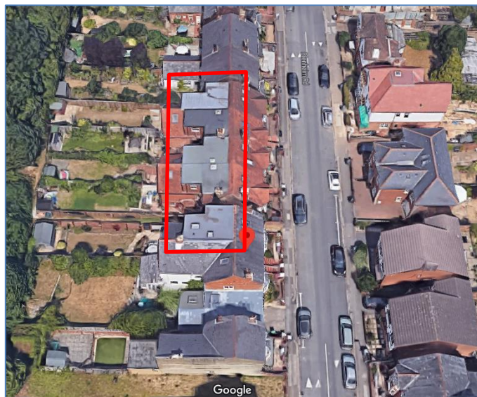
1. Examples of similarly design flat roof dormers along Blenheim Road.
