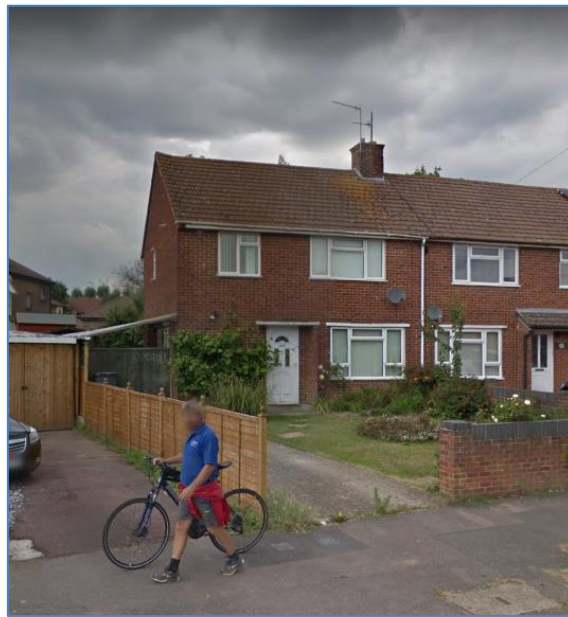
Fig 2. Google Street View image of the front of 260 Gainsborough Road. Image captured in July 2019.
