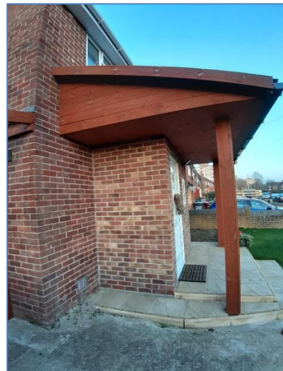
Fig 4. Side of 260 Gainsborough Road. Site photo provided by applicant on 09/12/2020.
