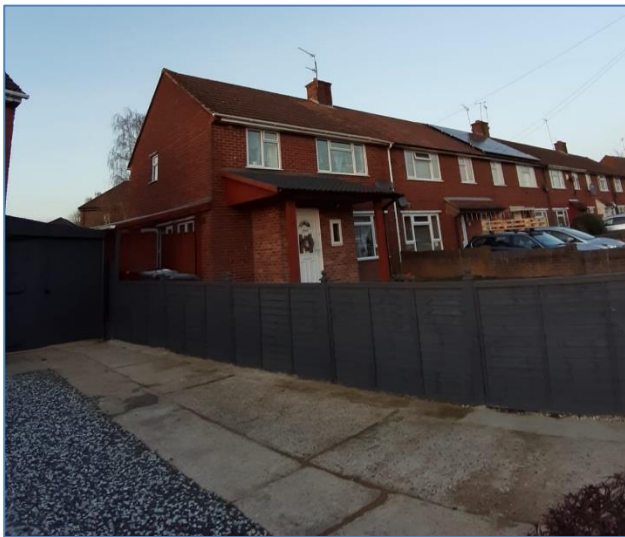
Fig 3. Front/Side photo of 260 Gainsborough Road. Photo supplied by applicant on 09/12/2020
