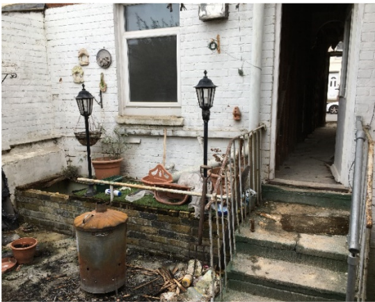
Existing light well and access from No.35
