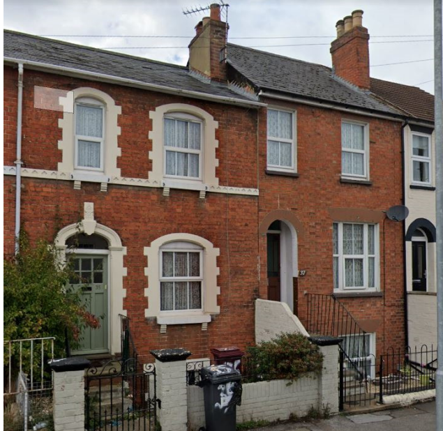
1. Front elevations of 35 and 37 Bedford Road houses.
