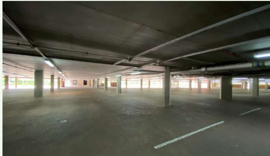
BASEMENT CAR PARK
