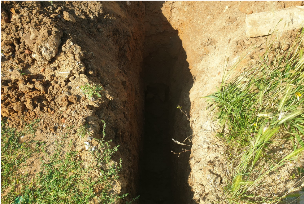
Photo from trial pit SA2
