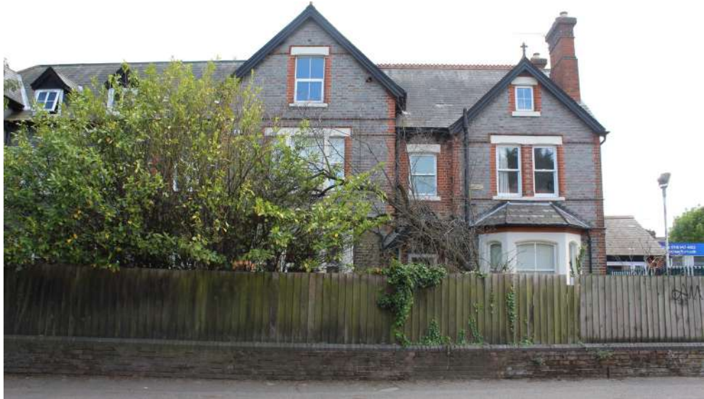
I Send Road - North Elevation exhibits qualities of Victorian houses
