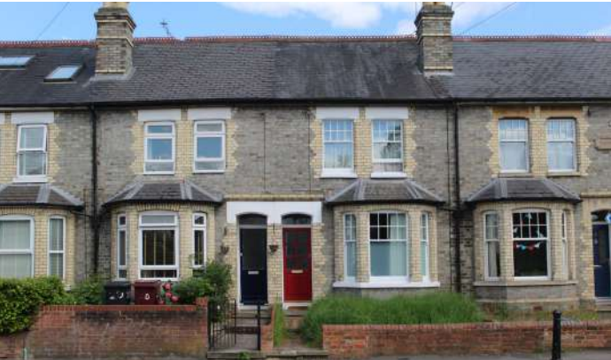
Example fenestration locally. Vertical paired windows and vertical windows to bay.
