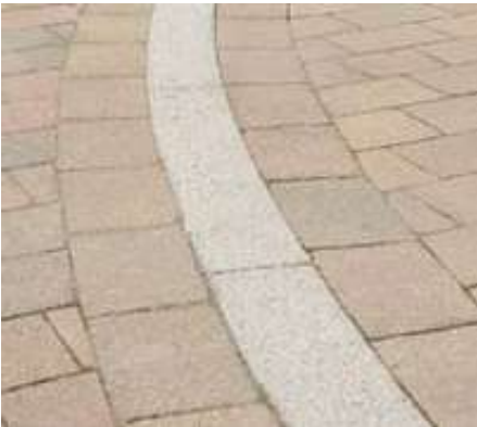
Flush granite style kerb to car park area - Marshalls Conservation kerb; silver grey colour
