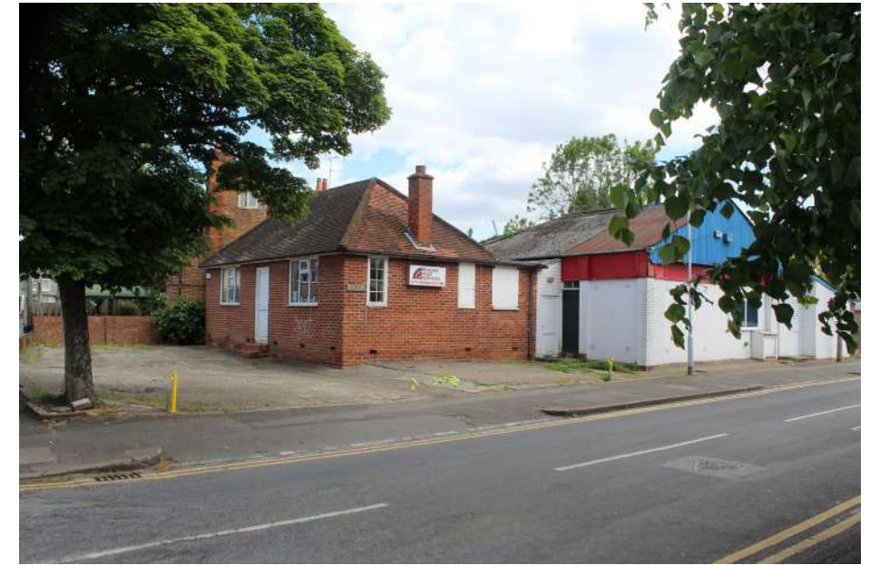
Existing vacant commercial building which provides no street presence
