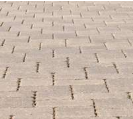
Permeable paving to car park area - Marshalls tegula priora; traditional colour
