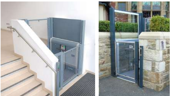
Example platform lifts
