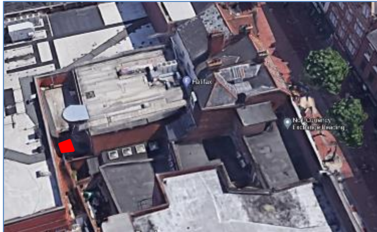
Fig 1. Aerial image of 65-67 Broad Street (submitted within the Design, Access & Planning Statement). The area in red demonstrates the location of the proposed air condenser unit.
