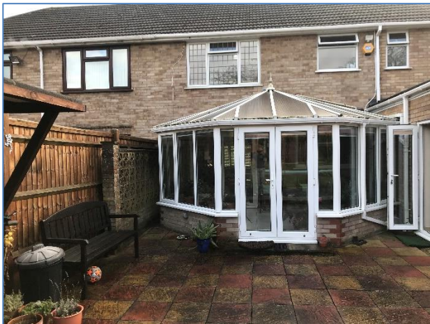
1. Rear of 58 Southcote Lane and side boundary to number 56. Photo provided by the agent on 04/01/2021.
