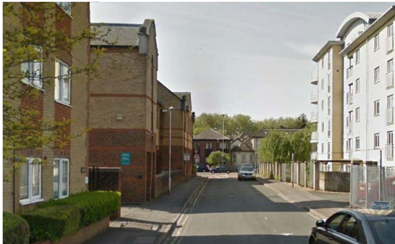
03. The Site. View from Rupert Street
