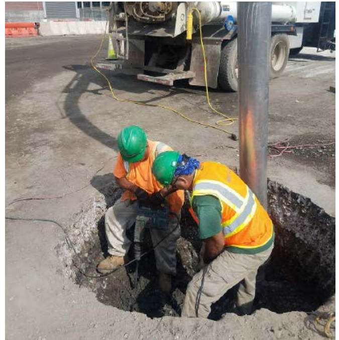
Vacuum excavation. Image: MTA Capital Construction
