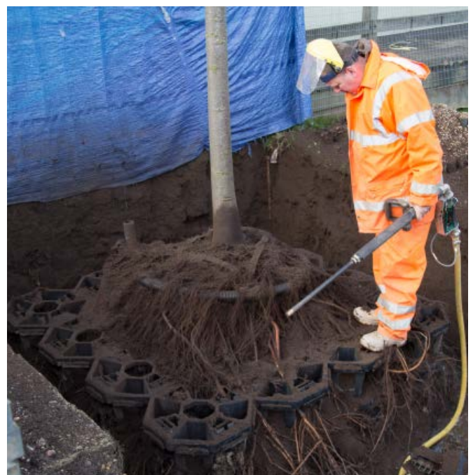
Tree pit excavation using air spading to prevent root damage.
