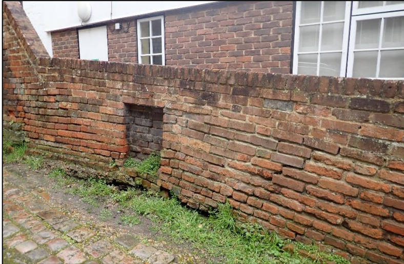
Figure 12. General view of the middle section of wall.
