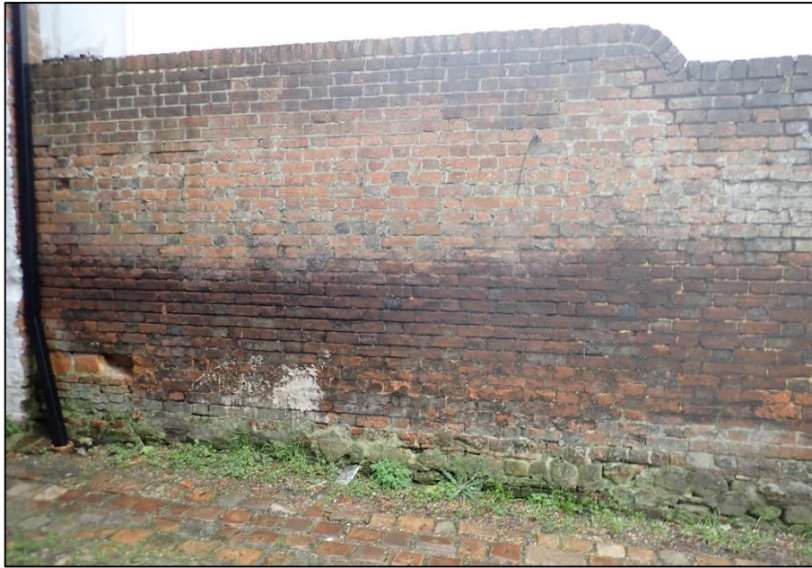
Figure 8. General view of the upper section of wall
