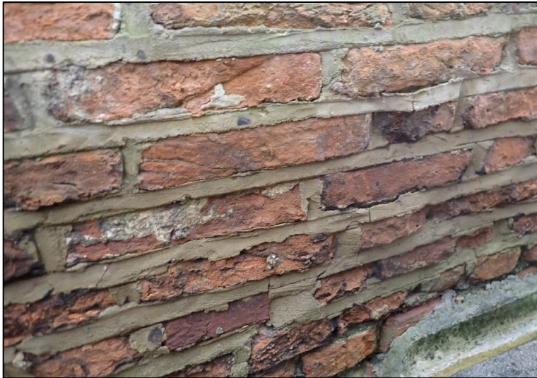
Figure 16. Cementitious pointing on the east side of the middle section of wall.
