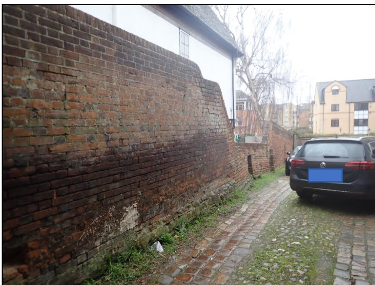
Figure 1. Partial view of wall (looking south from the carriage entry of No. 17)
