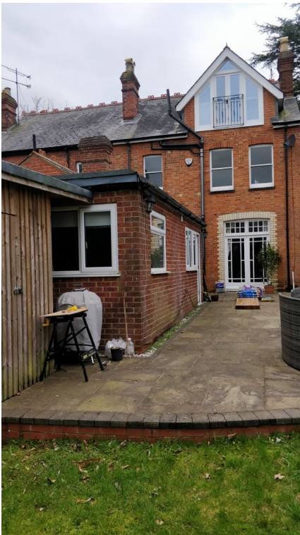
Rear of property showing existing extension
