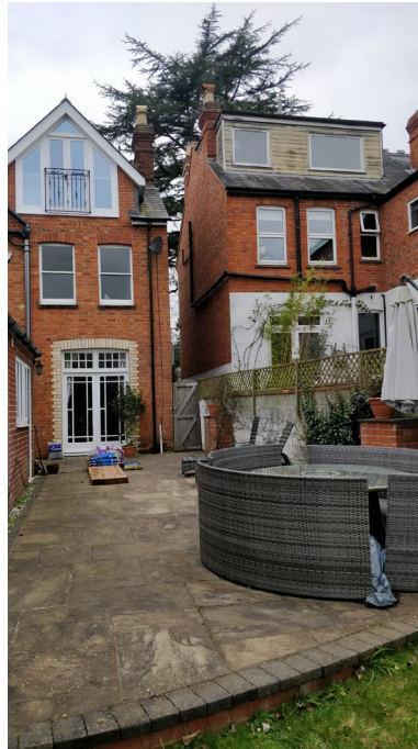
Boundary between 44 and 46 Priest Hill showing level difference between properties
