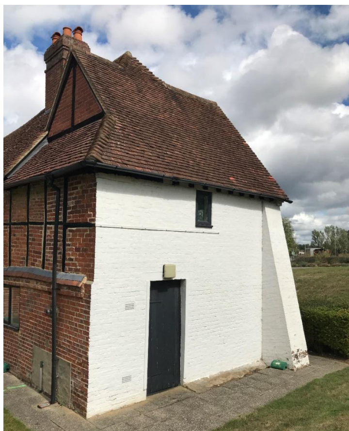
Figure 17 South elevation with gabled roof form
