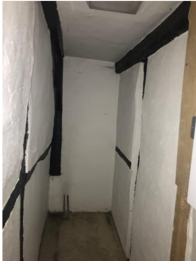
Figure 57 Storage room along west side of south first floor room.
