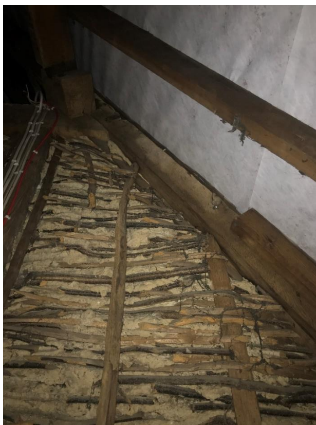
Figure 53 Wattle and daub partition in the attic space. The partition is above the wall between the central first floor room and the corridor to the south.
