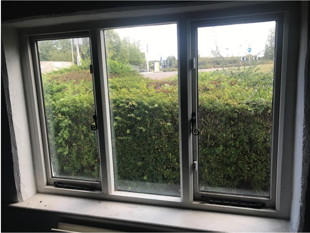
Figure 37 East window in north ground floor room.
