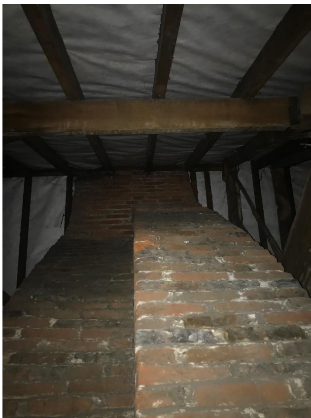
Figure 52 Looking up the brick chimney stack in the attic space above the corridor.
