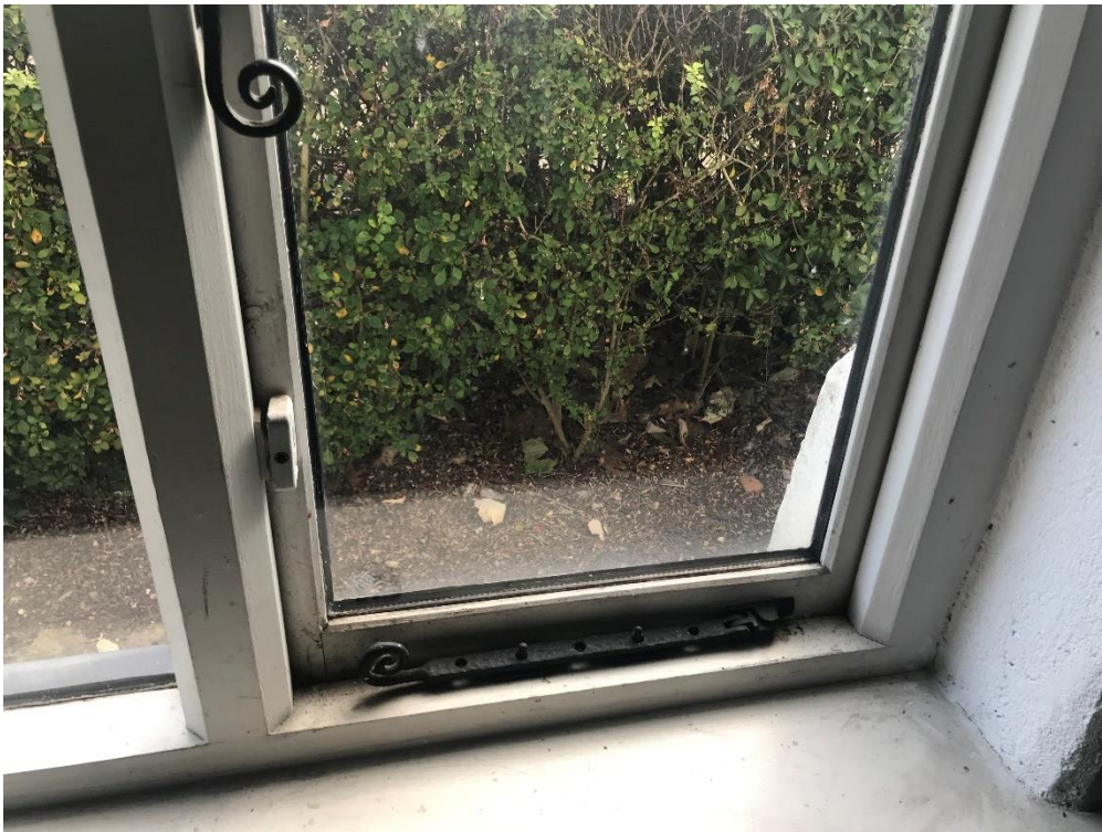
Figure 38 Detail of east window with curlicue stays in north ground floor room.
