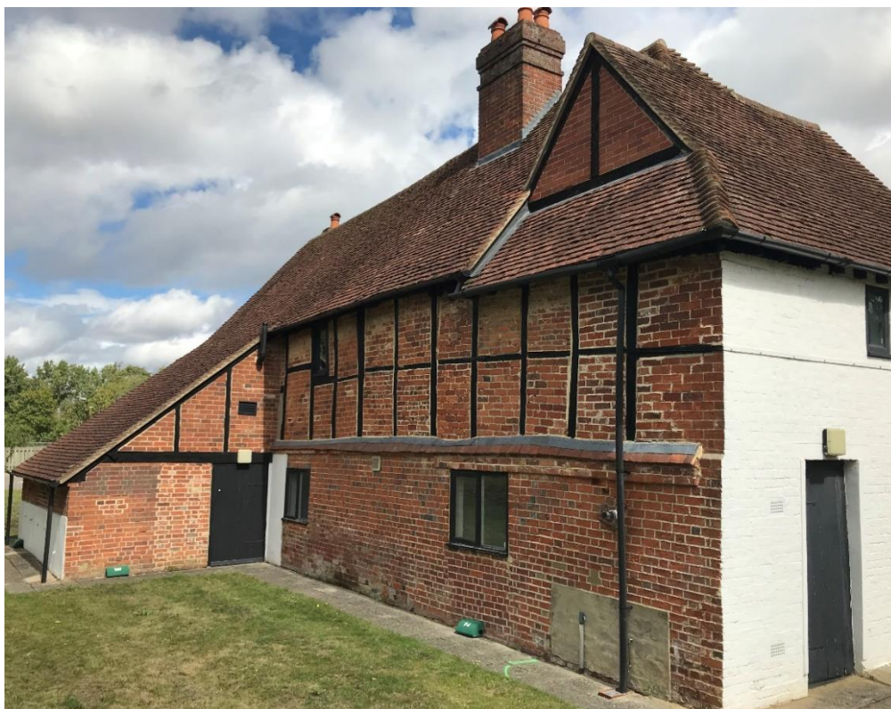
Figure 16 The rear (west) elevation, including the south side elevation of the catslide extension.
