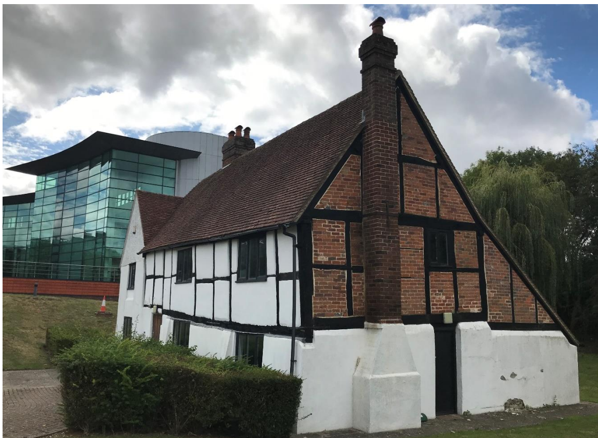
Figure 14 Looking towards the north gable end, including non-original external stack.
