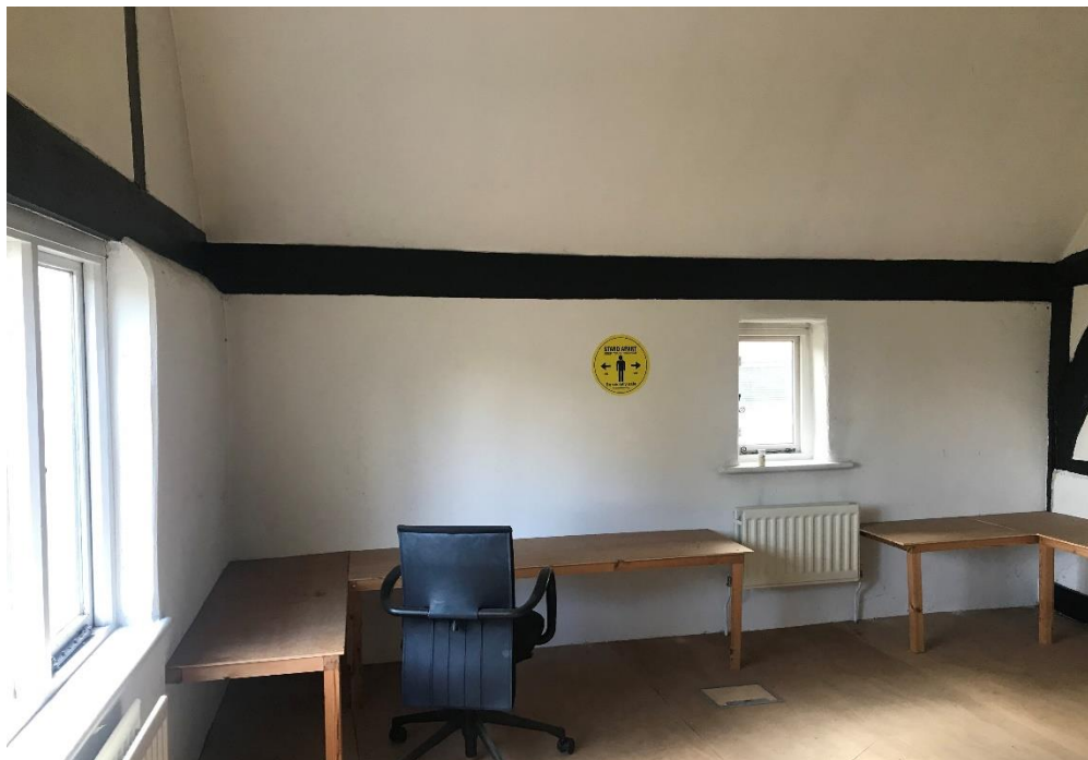
Figure 55 South end wall of south first floor room.
