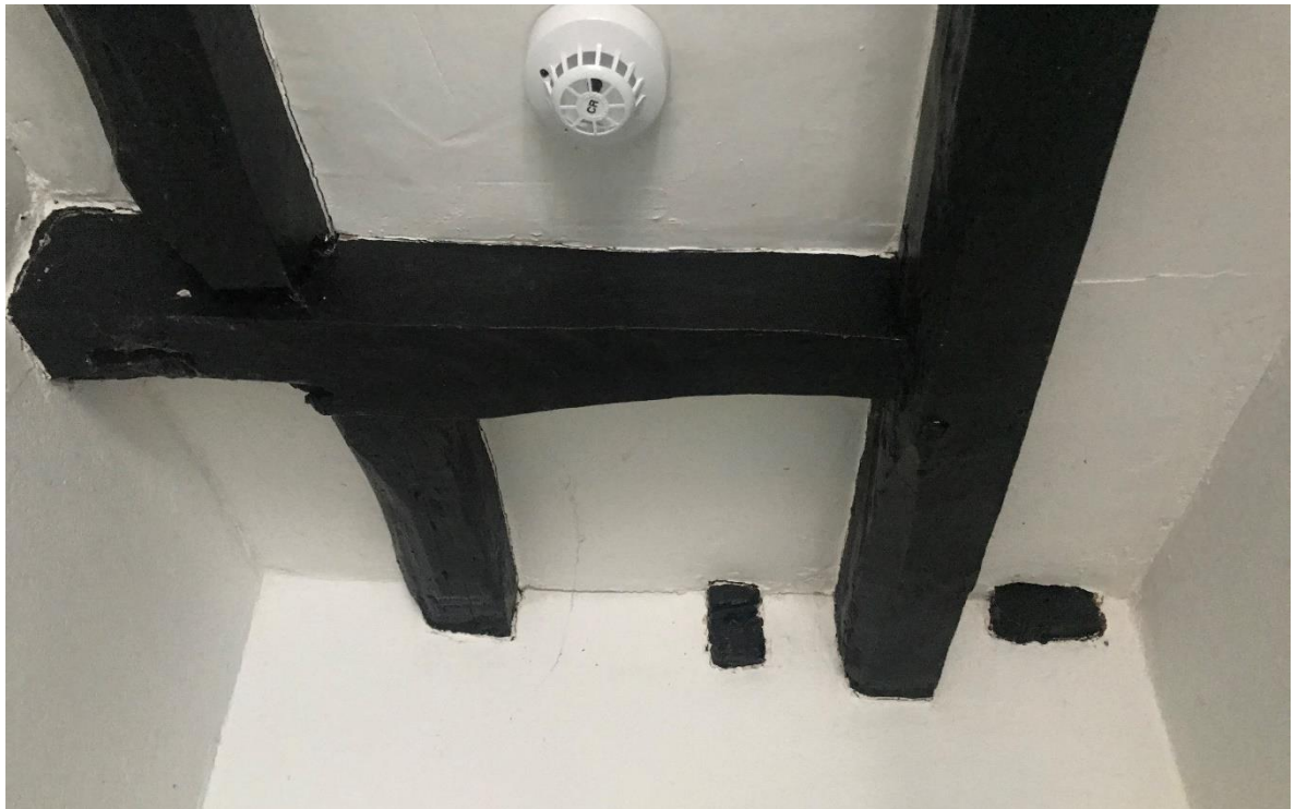
Figure 28 Adzed beams in the ceiling of the kitchen.
