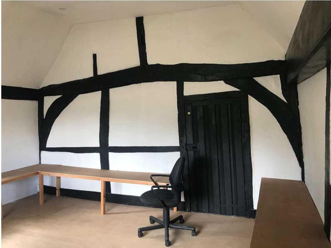
Figure 56 West wall of south first floor room. Historic timber door leads to the narrow room along the west side of the room.
