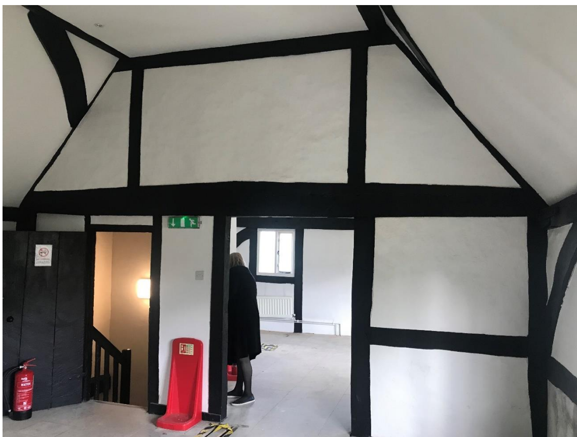
Figure 46 North wall of central first floor room.
