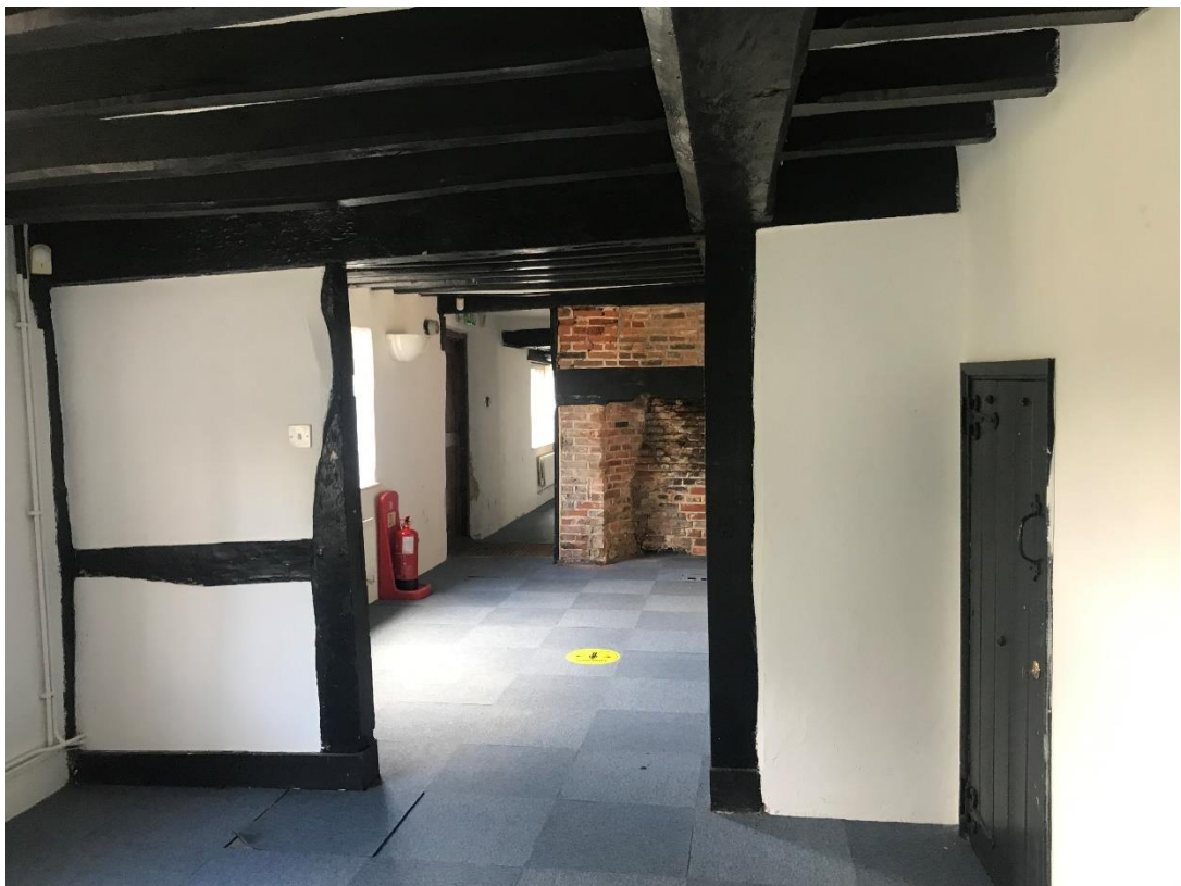
Figure 34 Looking south in north ground floor room.
