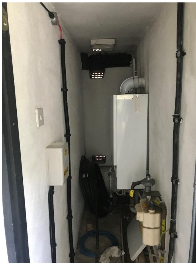
Figure 21 Storage room in the west of the south ground floor room.
