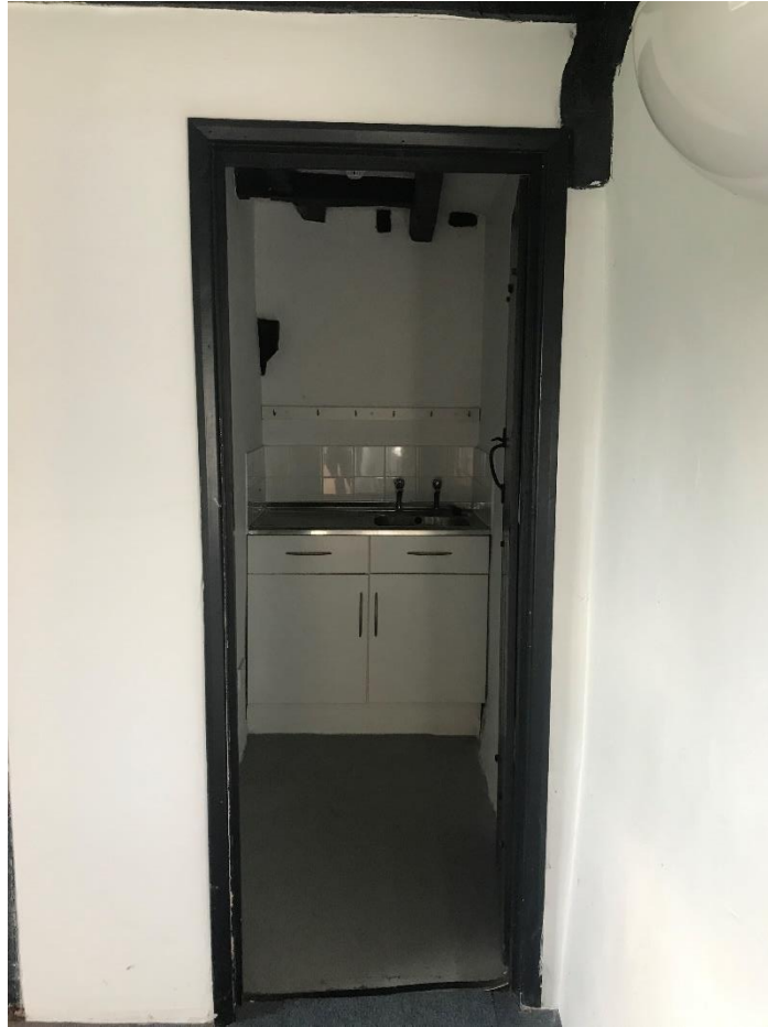
Figure 27 Kitchen to the north of the chimney stack to the west of the central room.
