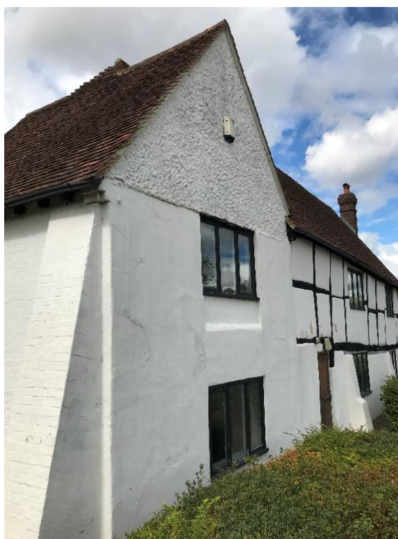
Figure 13 South-east corner of the building, including the cross wing.
