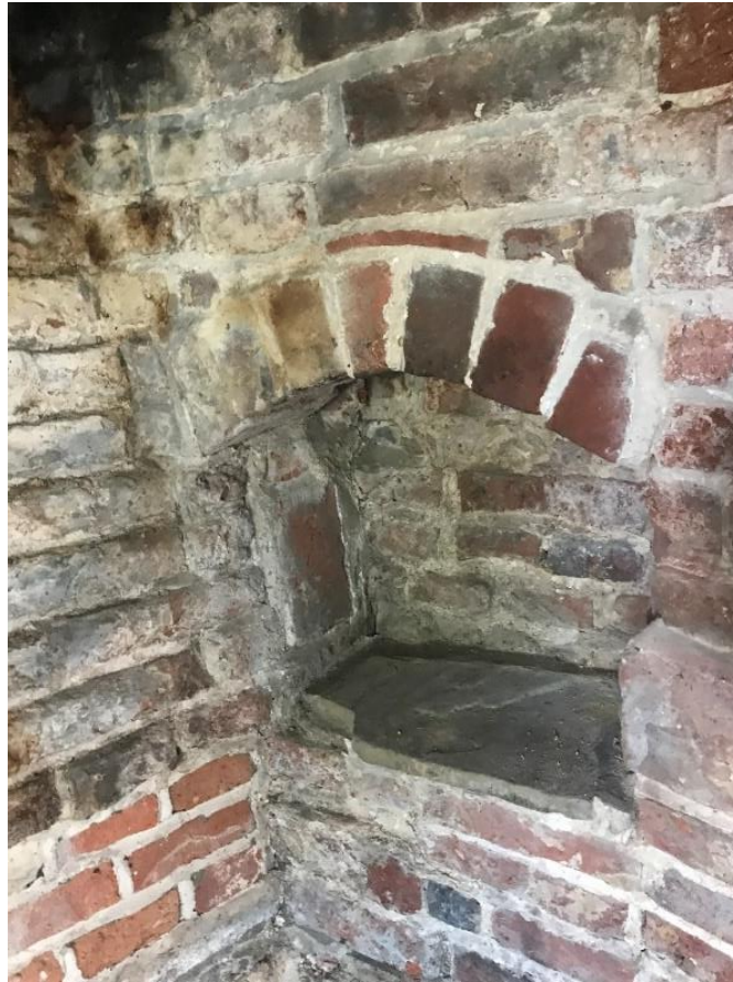
Figure 25 Niche in the side of the fireplace in the central ground floor room.
