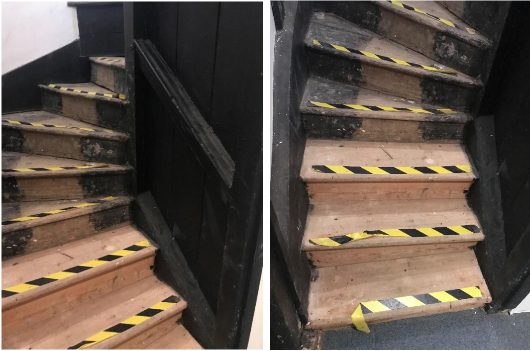
Figure 41 Stairs to the north-west of the central room.
