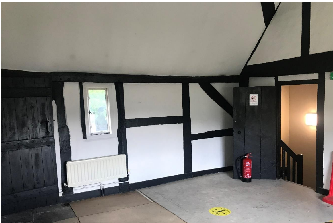
Figure 45 Looking west in the central first floor room. The top of the staircase is visible in the north-west corner (right).
