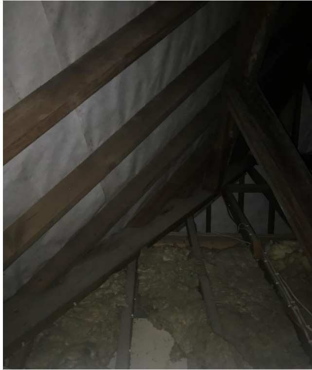
Figure 54 Partition above the north wall of the first floor corridor.
