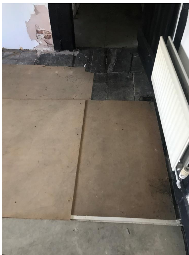
Figure 48 Modern boards over historic floor boards in central first floor room.
