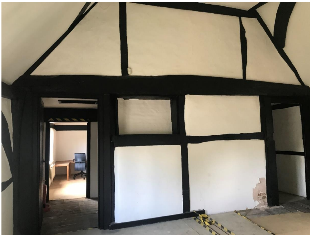
Figure 47 south wall of central first floor room.
