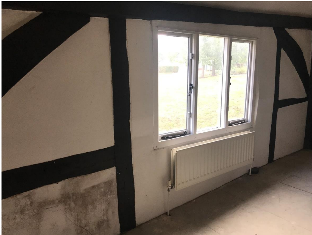
Figure 61 East wall of north first floor room.
