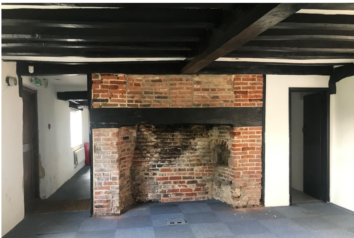
Figure 24 Fireplace in south wall of central ground floor room.
