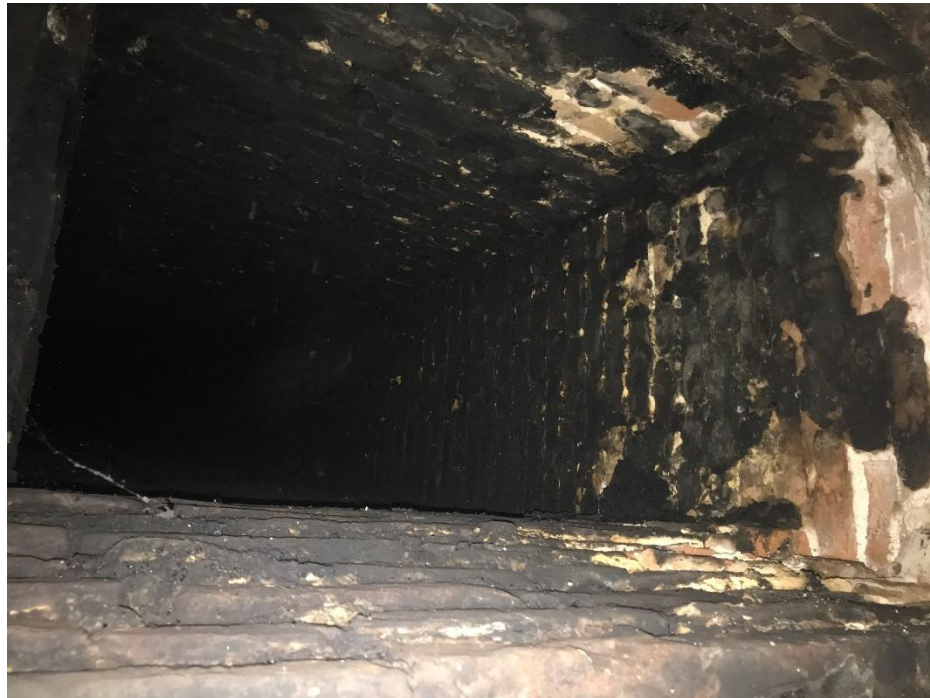
Figure 26 Looking up the flue from the fireplace in the central room.
