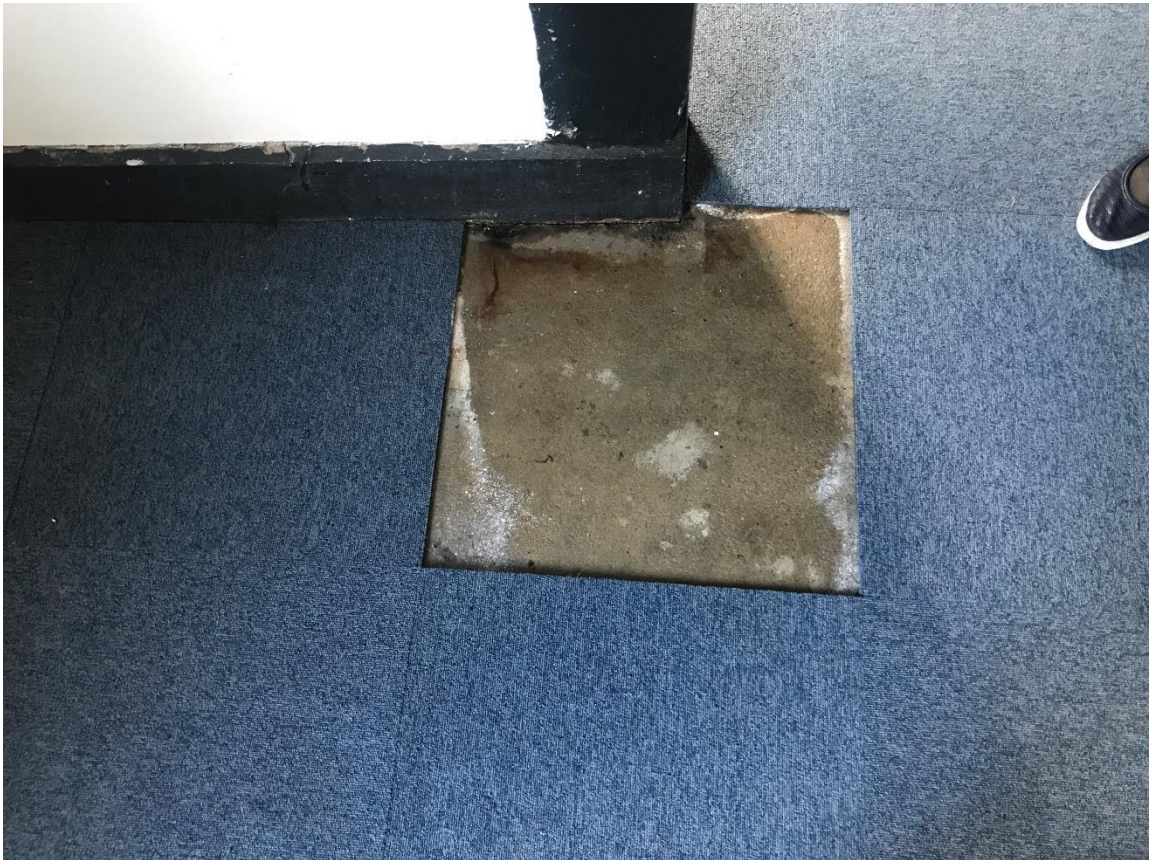
Figure 36 Concrete floor under carpet tiles in north ground floor room.
