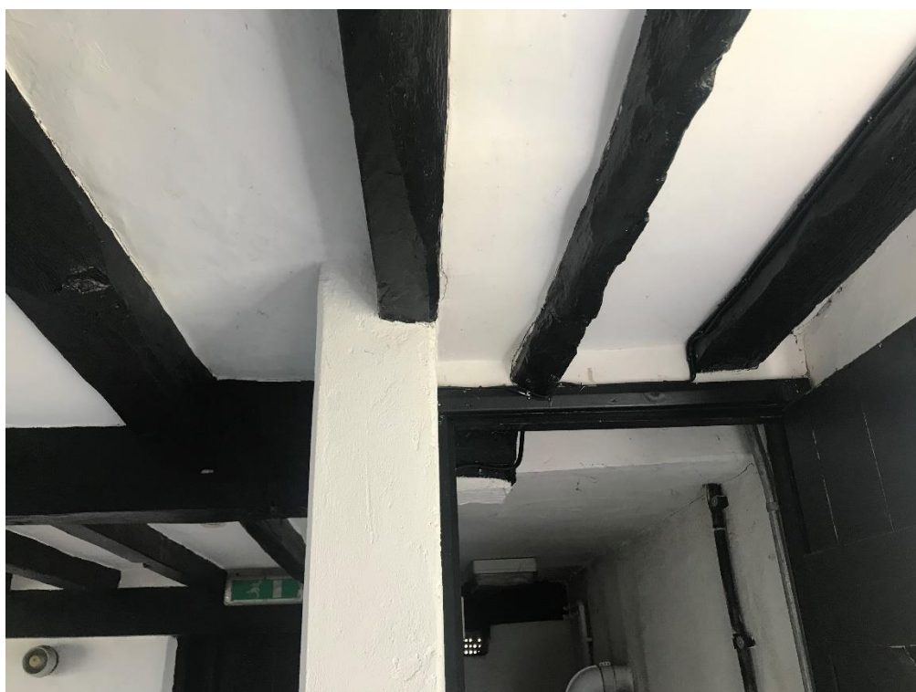
Figure 22 Ceiling of south ground floor room showing partition between the main room (left) and storage room (right).
