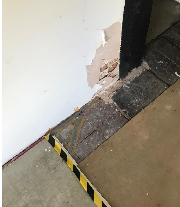
Figure 49 Modern boards in central first floor room. Clay tiles are visible in front of the south wall, suggesting a hearth.
