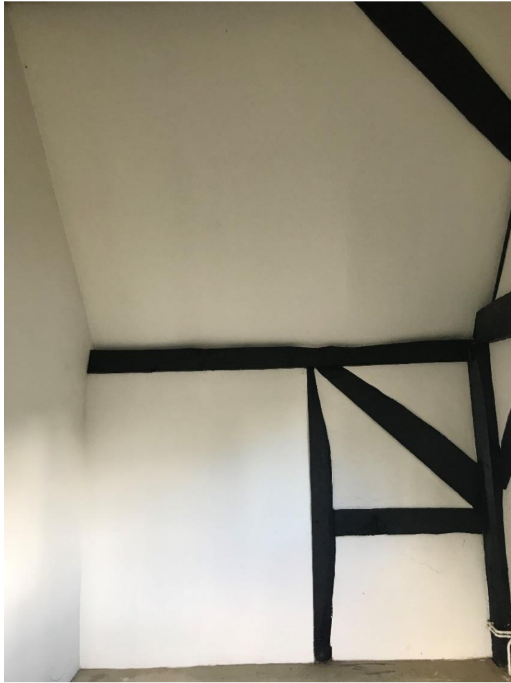
Figure 60 West wall and roof slope of north first floor room.
