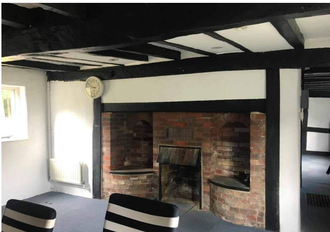
Figure 20 Fireplace in the north of the south ground floor room. The brick in-fill structures are not original.
