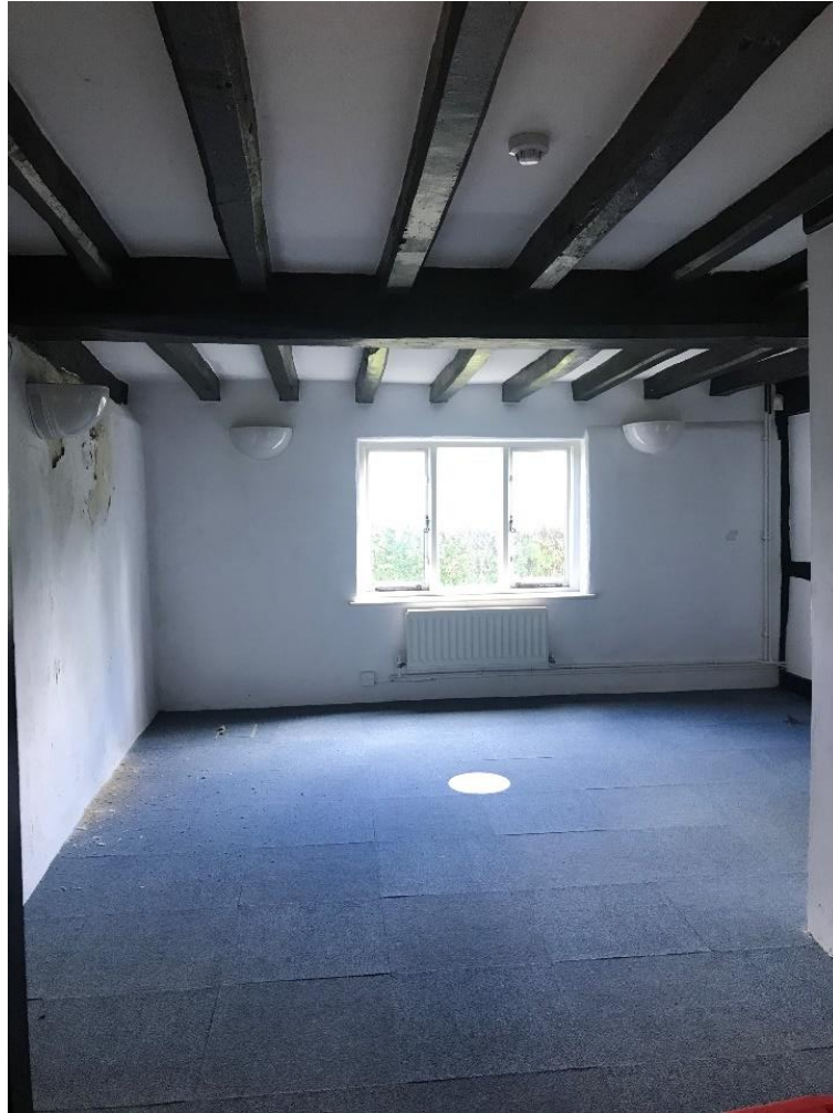
Figure 29 Looking east in north ground floor room.
