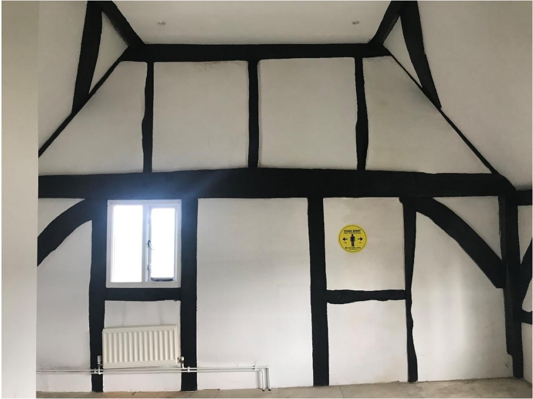
Figure 58 North wall of north room.
