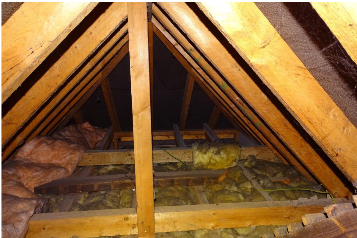
Image 11 – Section of the roof void which was restricted from access for inspection due to the position of the water tank. It was confirmed that a felt membrane covering was in place below the roof tiles
