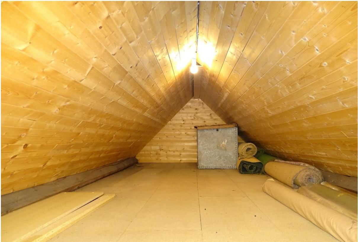
— Image 10 – Internal view from within the accessible section of the roof void space which has been cladded internally with timbers below the felt membrane coverings
