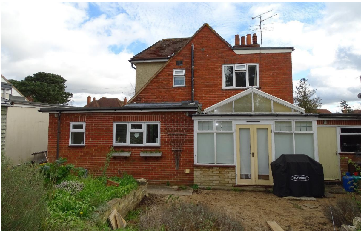
Image 4 – Rear West facing elevation of the property
