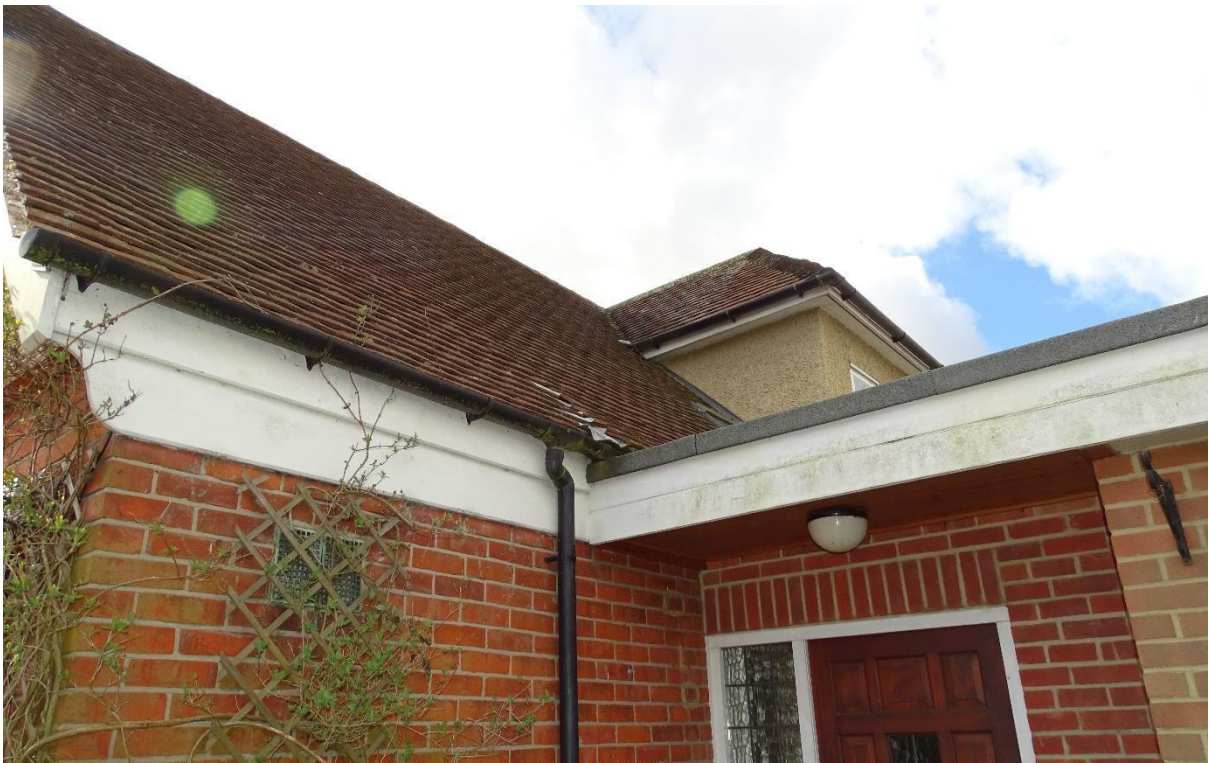
Image 3 North facing roof coverings
