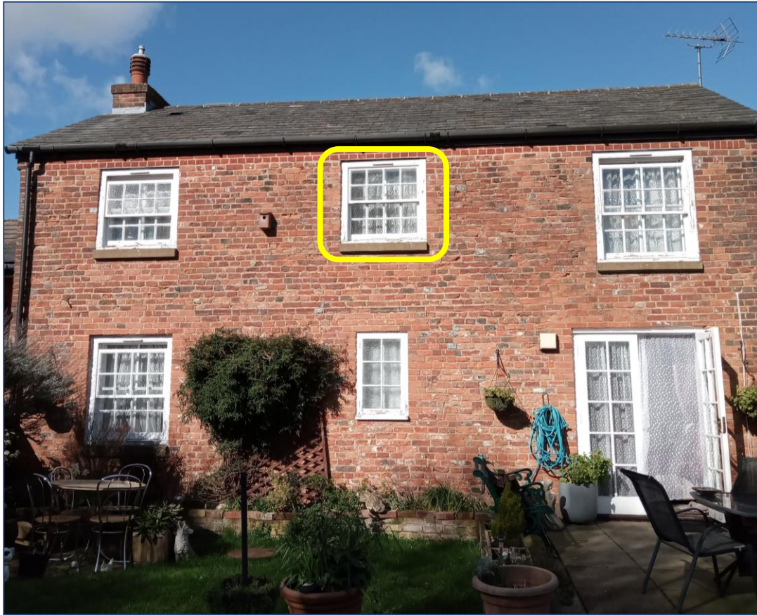
1. Window to be replaced highlighted in yellow box.
