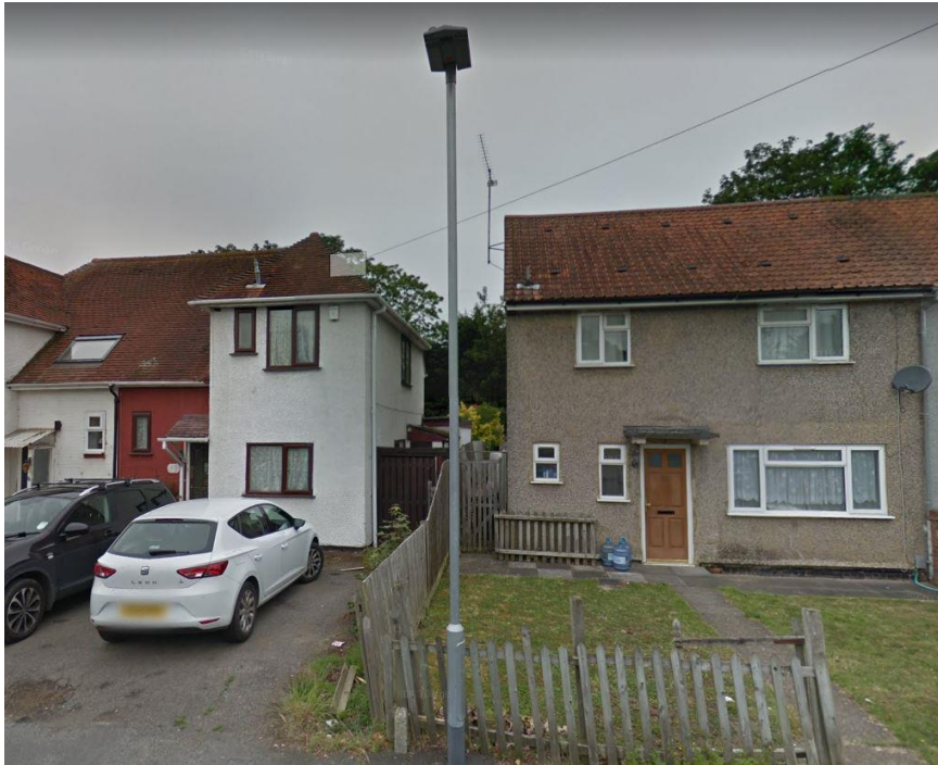
Relationship of No. 4 (left) and No. 170 Linden Road (which are identical house types).
