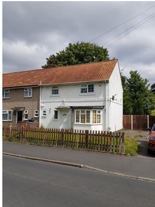
No. 9 and No. 7 showing current Built form of Terrace Block
