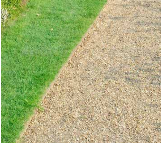
Timber edging along footpath
