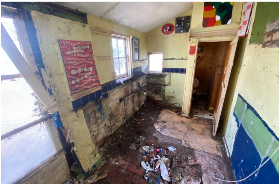
Fig.8 Interior view of existing rear extension G-05
