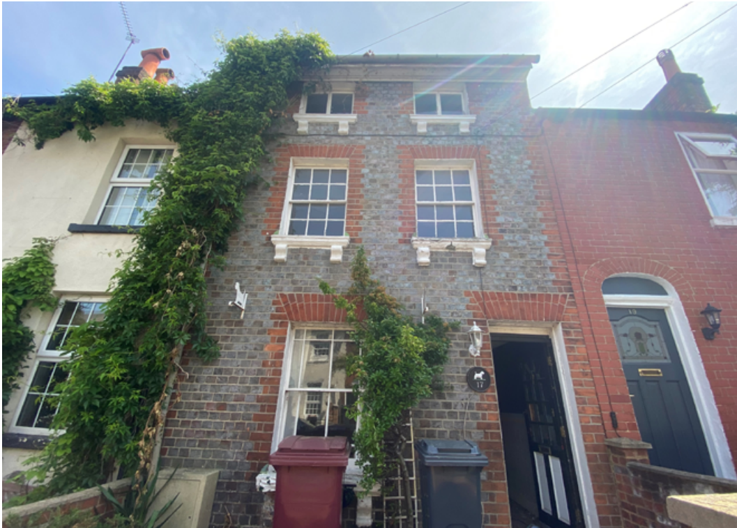
Fig.1: Existing view of 17 St Johns Street facade
