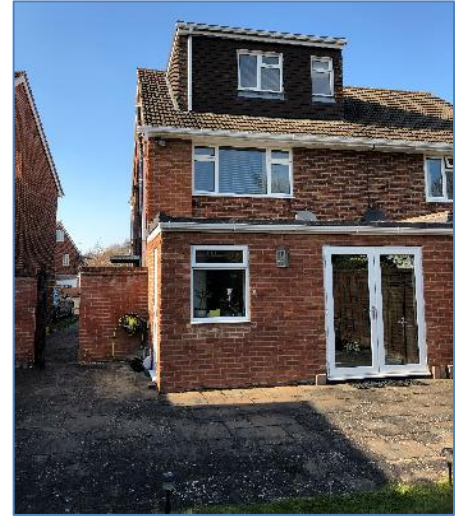
5. Rear Elevation of 20 Vine Crescent - photo provided by agent on 22/06/2020.
