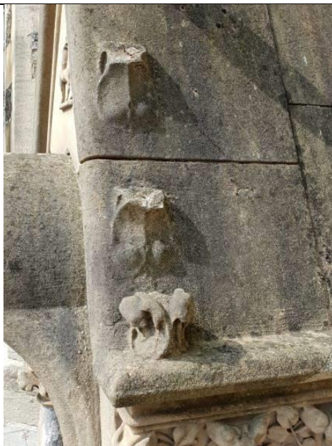
Fig 8. Decorative carved details that need to be reinstated. Cut out and or pinned in place as stated in repair schedule. (RBC. 2020)
