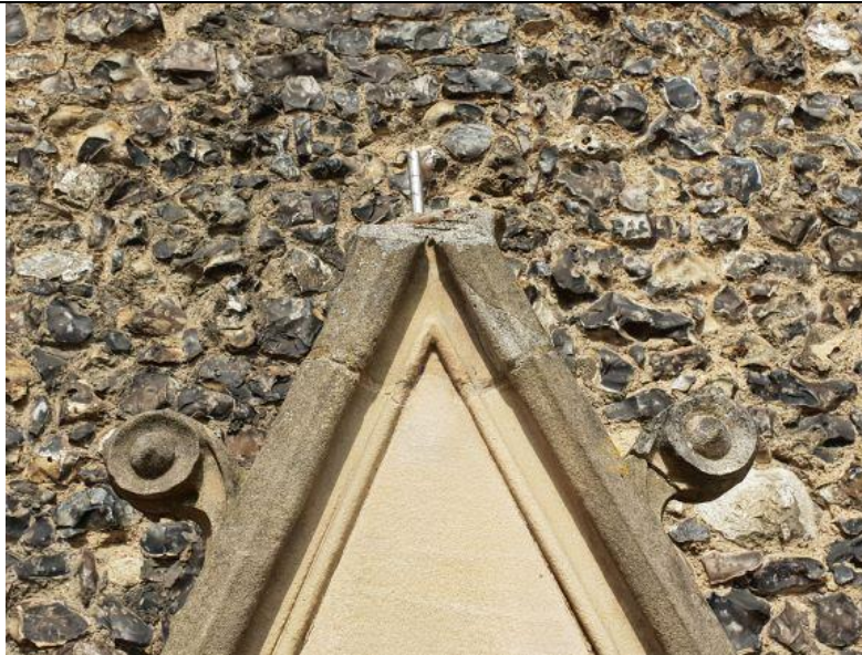
Fig 7. Missing top finial stone details missing. (RBC. 2020)
