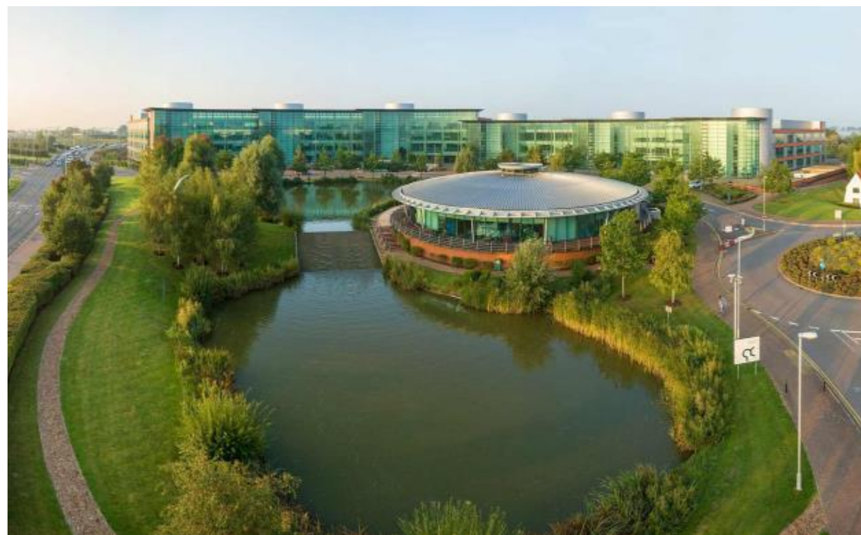
Existing Site View
