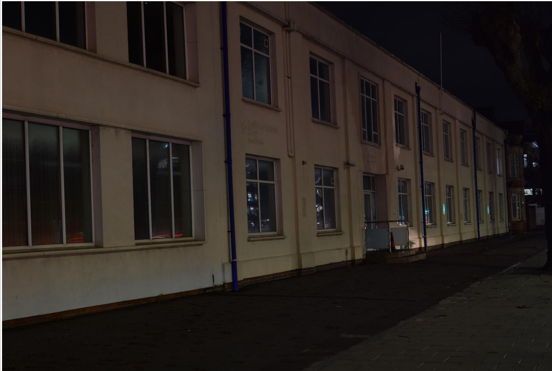
F - View the southern site boundary from Vastern Road
