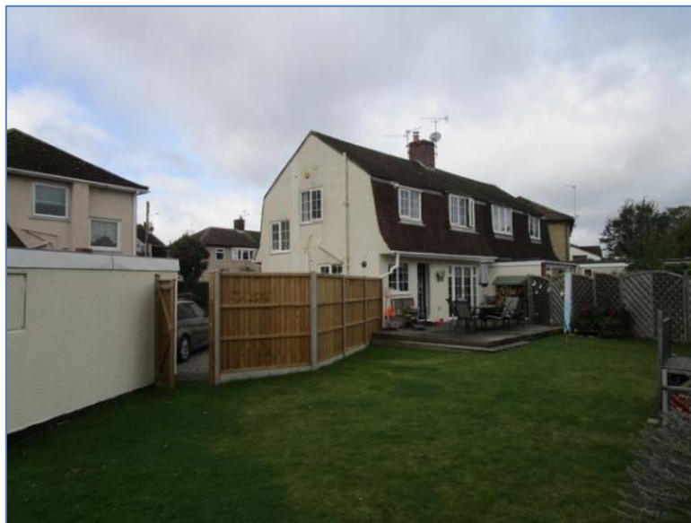
Fig 2. Rear/Side elevation. Site photo provided by agent on 07/12/2020.
