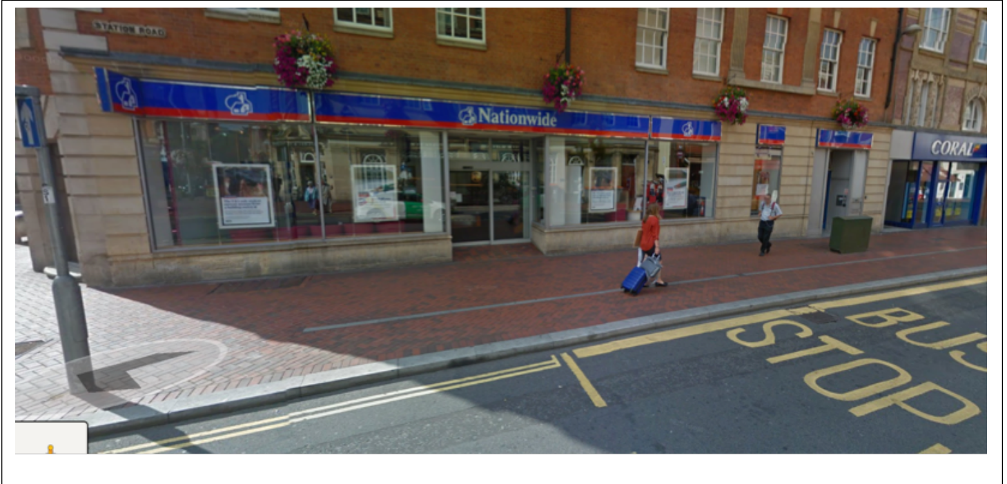
Former Nationwide Station Road shopfront:
