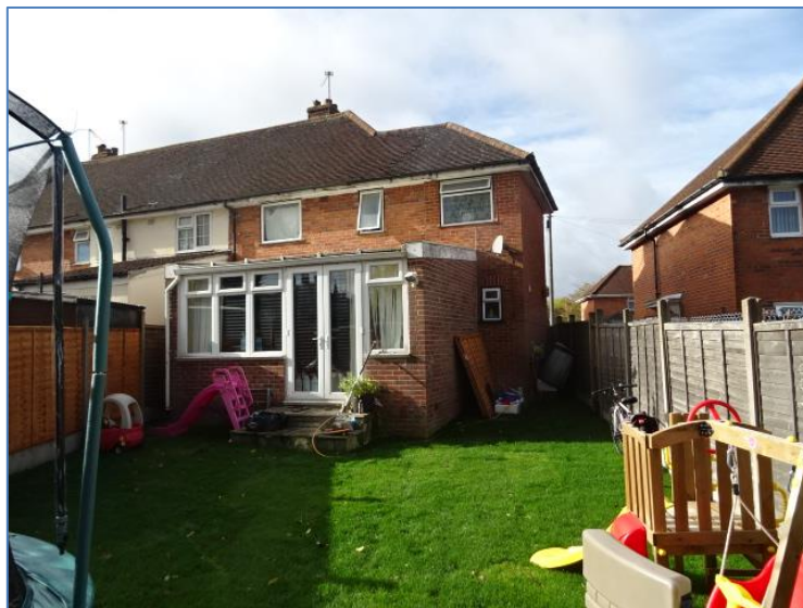
Fig 1. Rear of 27 Lamerton Road. Site photo provided by agent on 16/12/2020.
