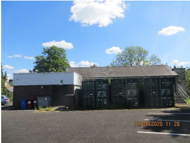
Photo 2 – View of the rear Elevation
