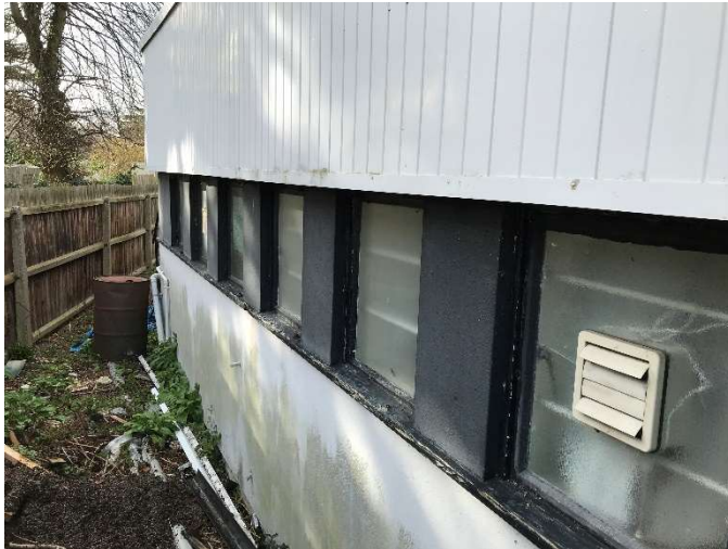
Photo 5 – View to the rear of the existing toilets
