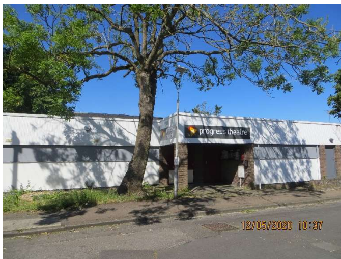
Photo 1 – View of the front elevation (with permission the tree has been removed since this photo was taken)
